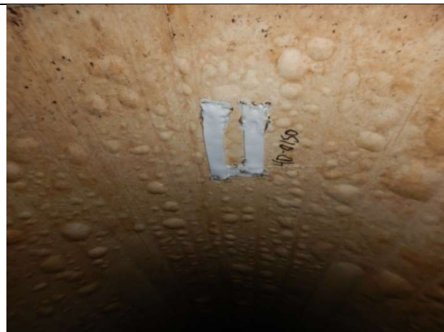
Liner repair at the crown (12:00)
