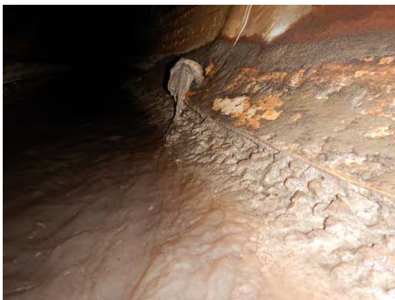
Photo 3-11. Typical exposed aggregate in channel.
