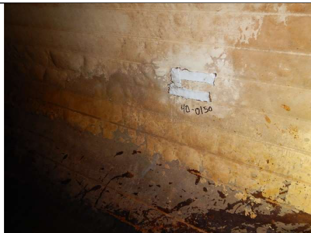
Liner repair at spring line (3:00)
