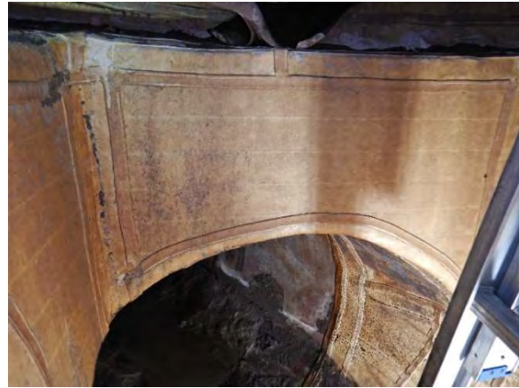
Photo 3-10. Typical termination at pipe and MAS interface.
