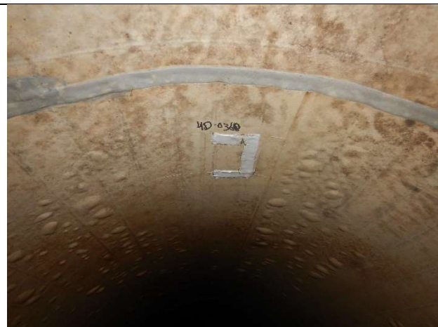
Liner repair at the crown (12:00)
