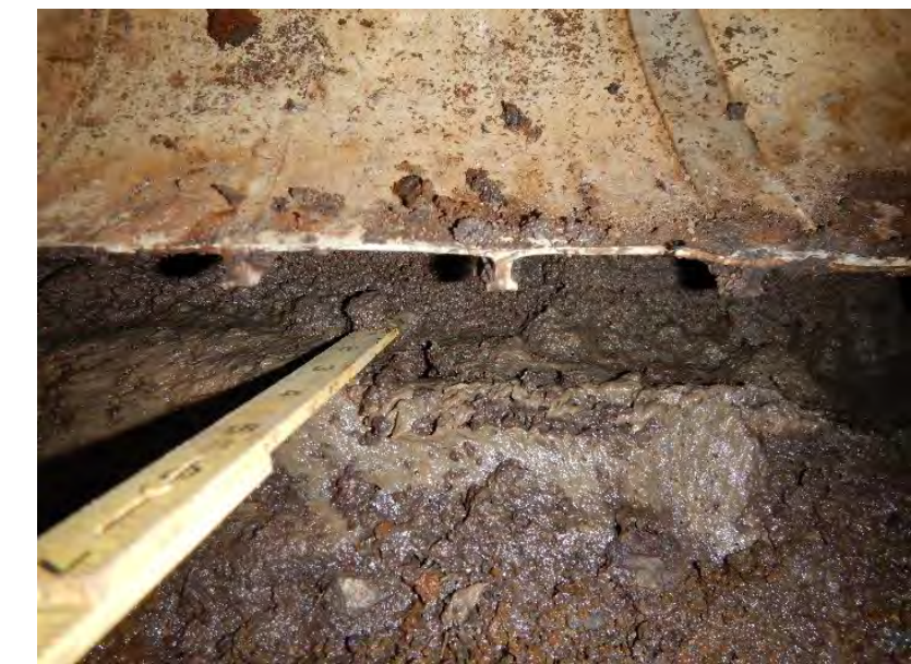
Figure 2: Unlined concrete testing
