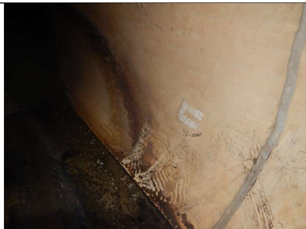
Liner repair at spring line (4:30)
