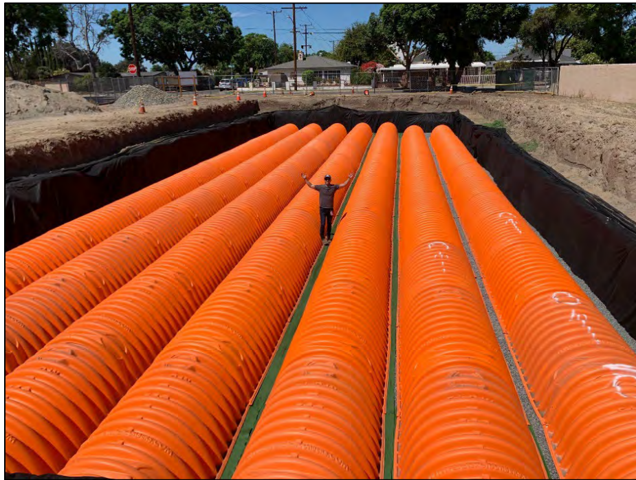
Subsurface infiltration system
