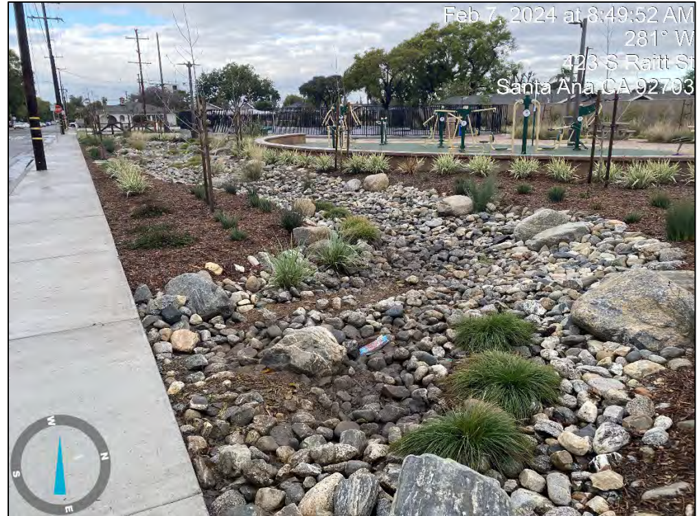
Bioretention Basin #2 (Post-Storm)
