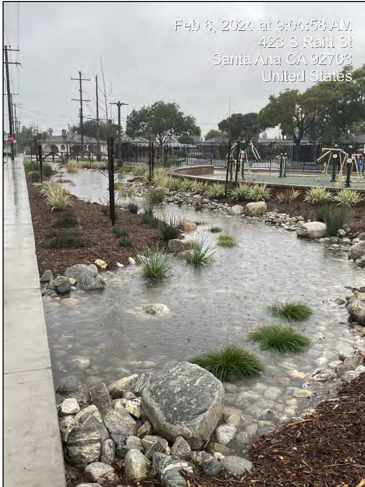
Bioretention Basin #2 (During Storm)
