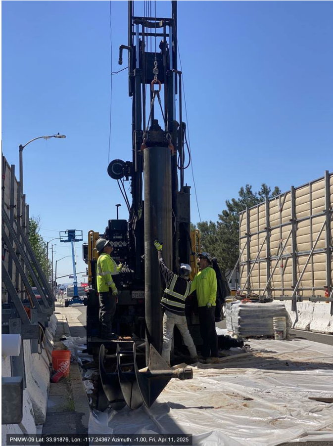
20 ft Conductor Casing Installation (PNMW-09)
