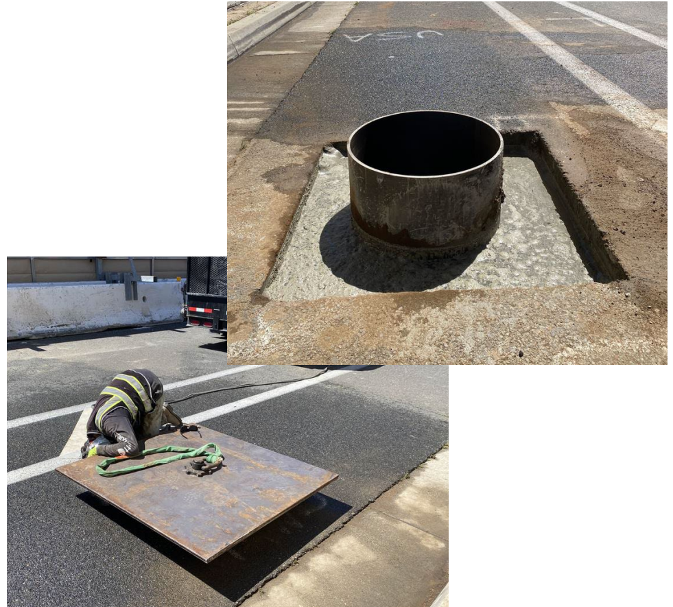
20 ft Conductor Casing Installation (PNMW-09)
