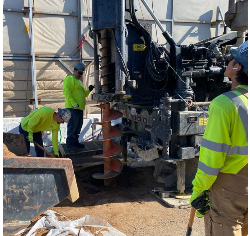
Drilling 32" Dia. Conductor Borehole (PNMW-08)
