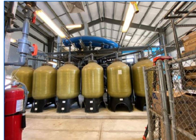
ISEP IX system provided by Calgon Carbon
