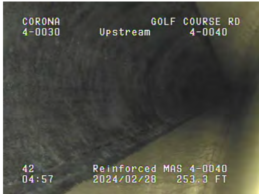
Figure 3: Typical Pipe Wall Condition
