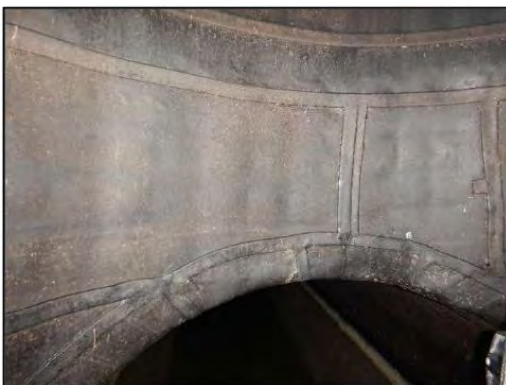
Figure 9: Typical Condition of Liner Weld Strips
