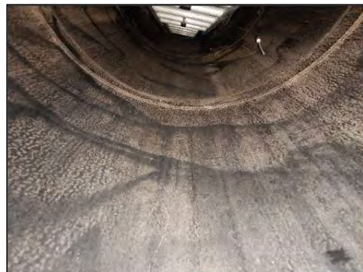
Figure 10: Typical Liner Condition
