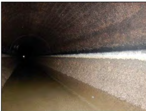
Figure 7: Typical Pipe Condition Typical Maintenance Access Structure Conditions
