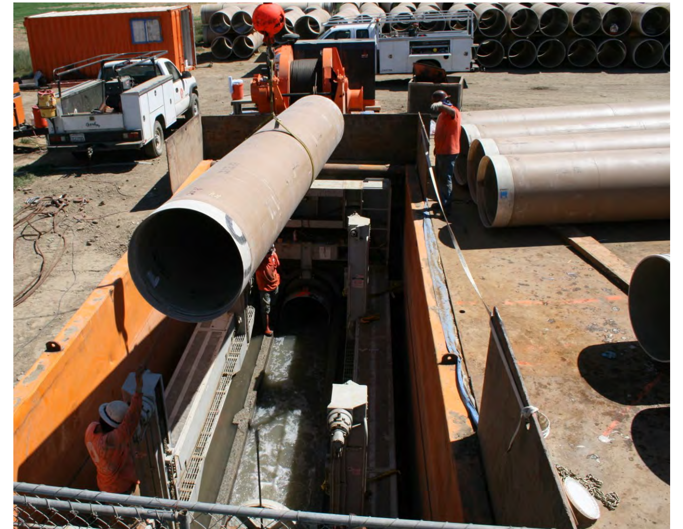
Reach IV-A and IV-B Rehabilitation Project
