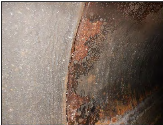
Figure 15: Lining Failure at U/S Joint
