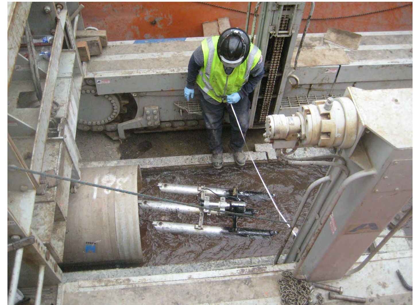
Reach IV-A CCTV Inspection
