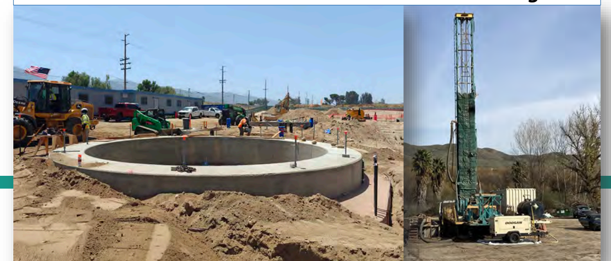
Elsinore Basin Wells GAC Backwash Foundation Well 2 Drilling
