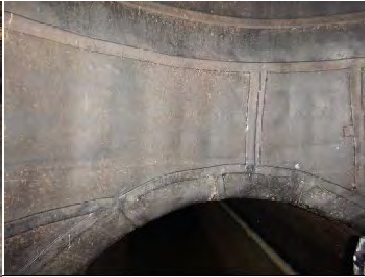
Liner Termination at influent pipe good condition
