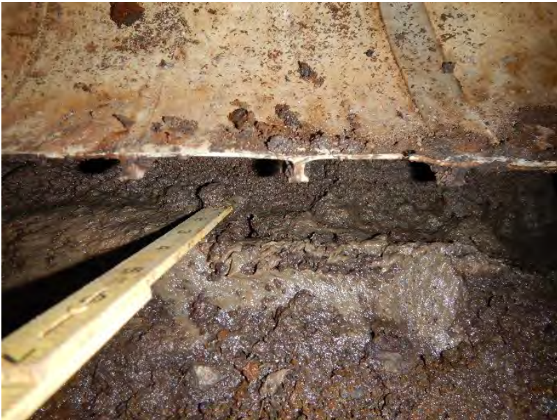
Figure 2: Unlined concrete testing
