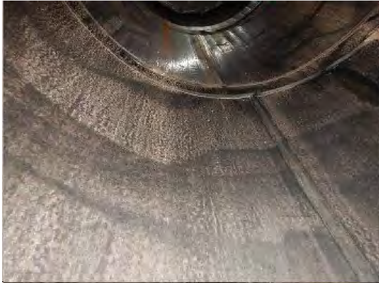
Interior of MAS in good condition
