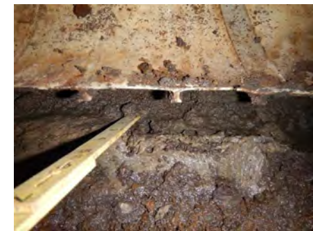
Figure 2: Unlined concrete testing
