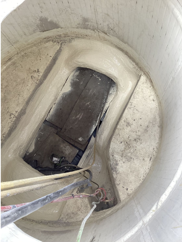
Figure 2: Coating applied to New Brine Line Connection MAS.
