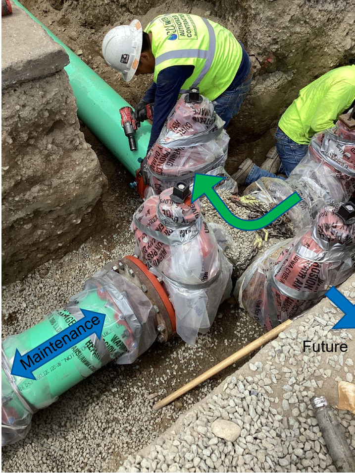
Figure 3: Cross connection to existing RBF Lateral.
