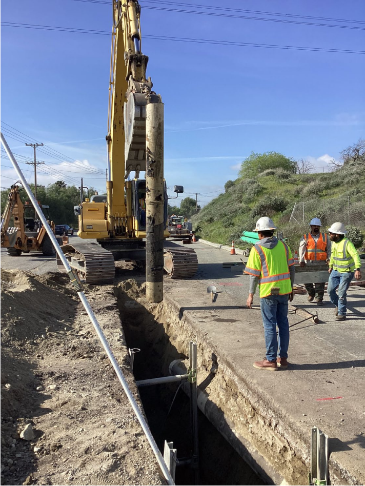
Figure 1: Removal of abandoned 12" steel pipe.
