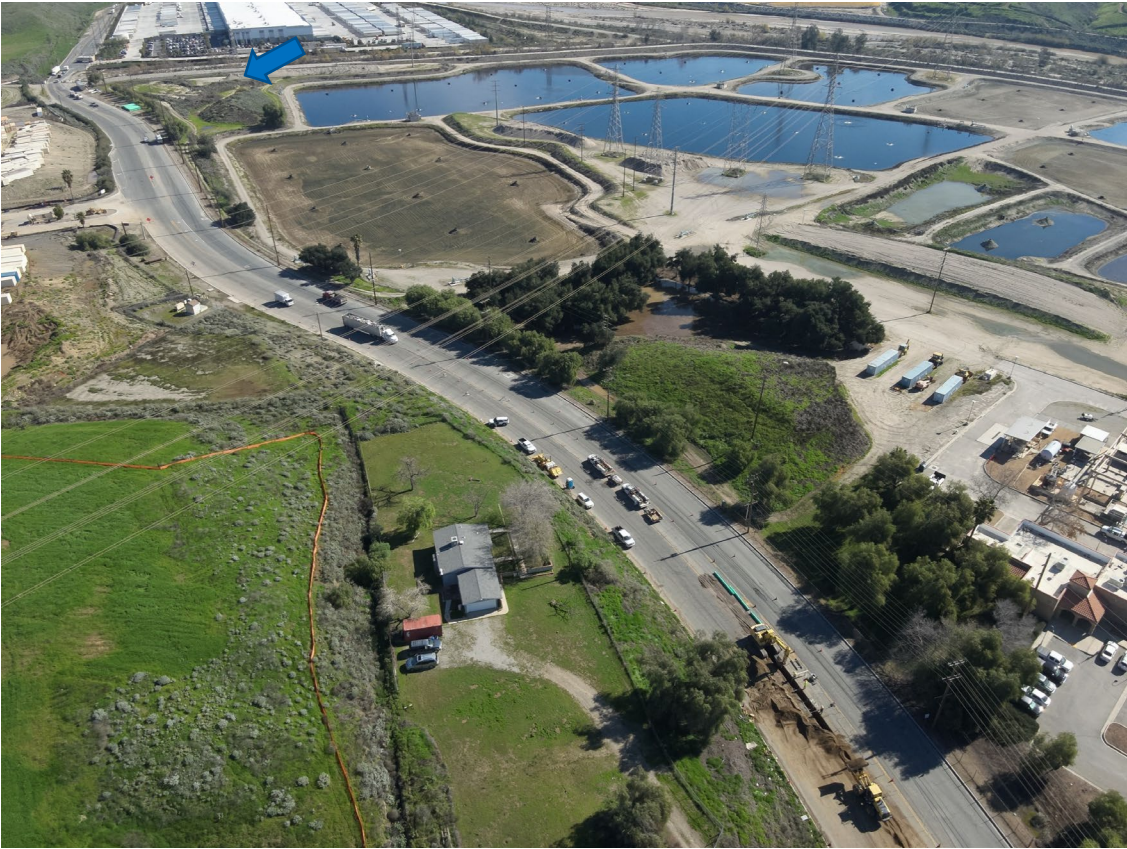
Figure 1: Looking East along Agua Mansa Road
