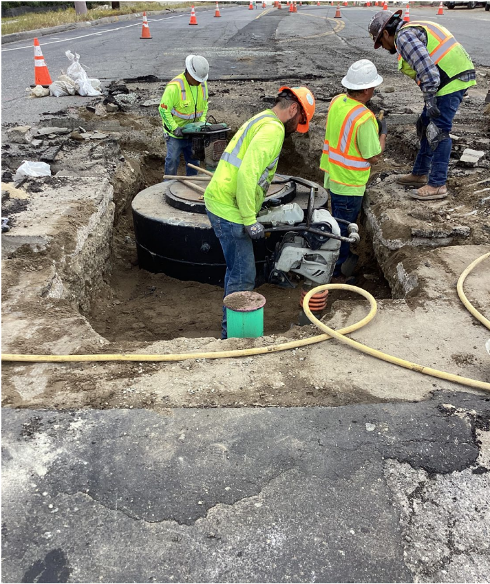
Figure 3: Backfill and compacting around new MAS
