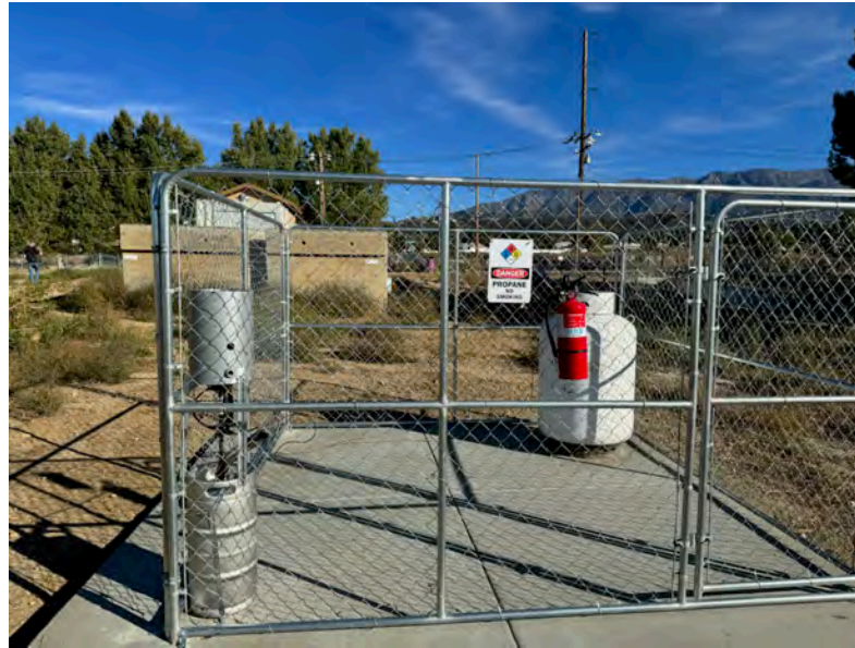
NE10: San Geronio Pass Water Agency
