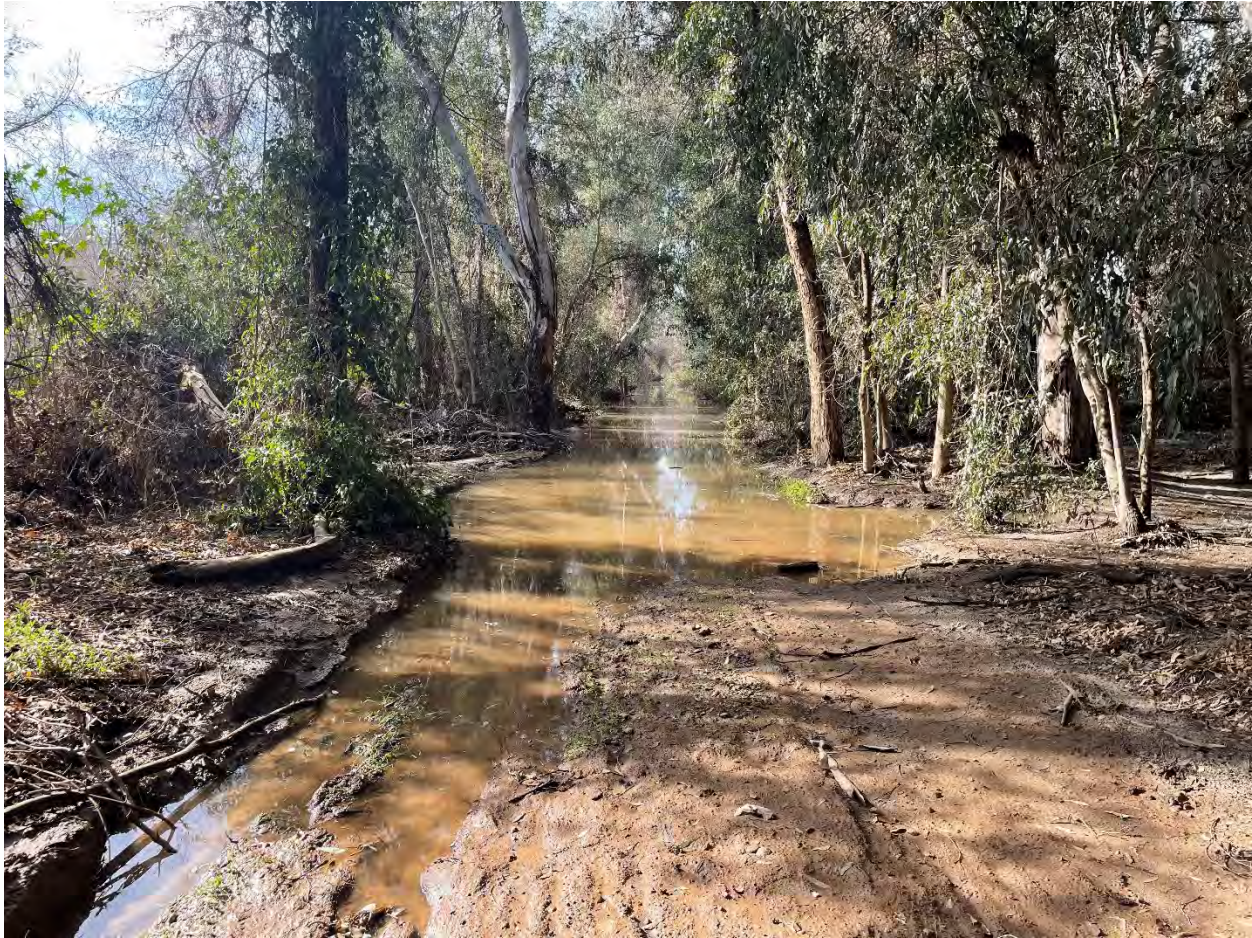
Figure 1 Image of Access Road conditions within the Prado Dam Inundation Area
