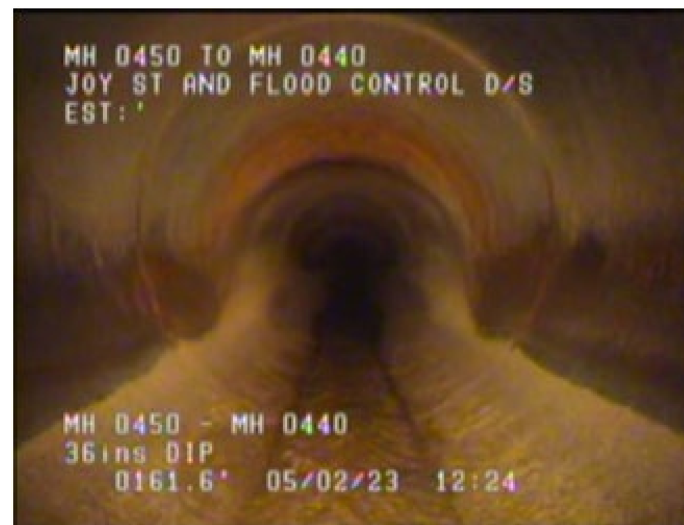
Corrosion Discoloration at Crown and Joint
