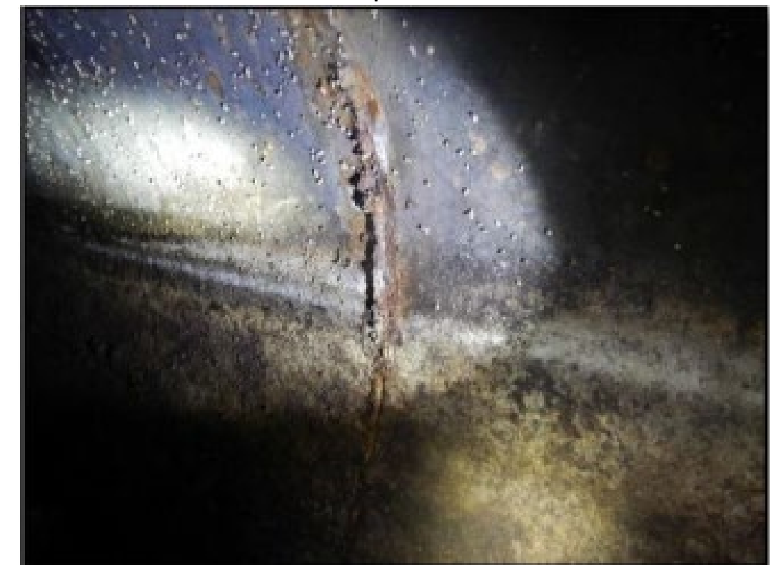
Coating Failure at Joint
