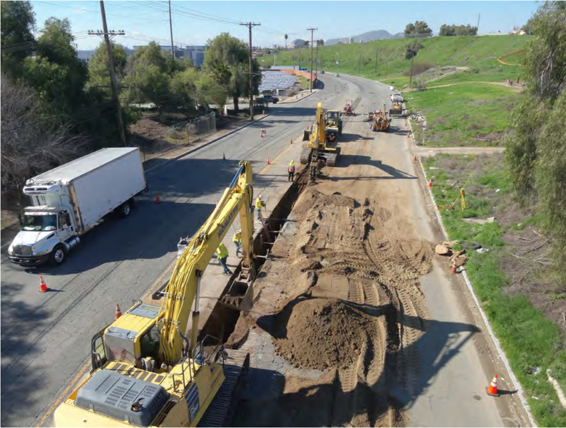
Figure 1: Excavation, installation and backfill of pipe.
