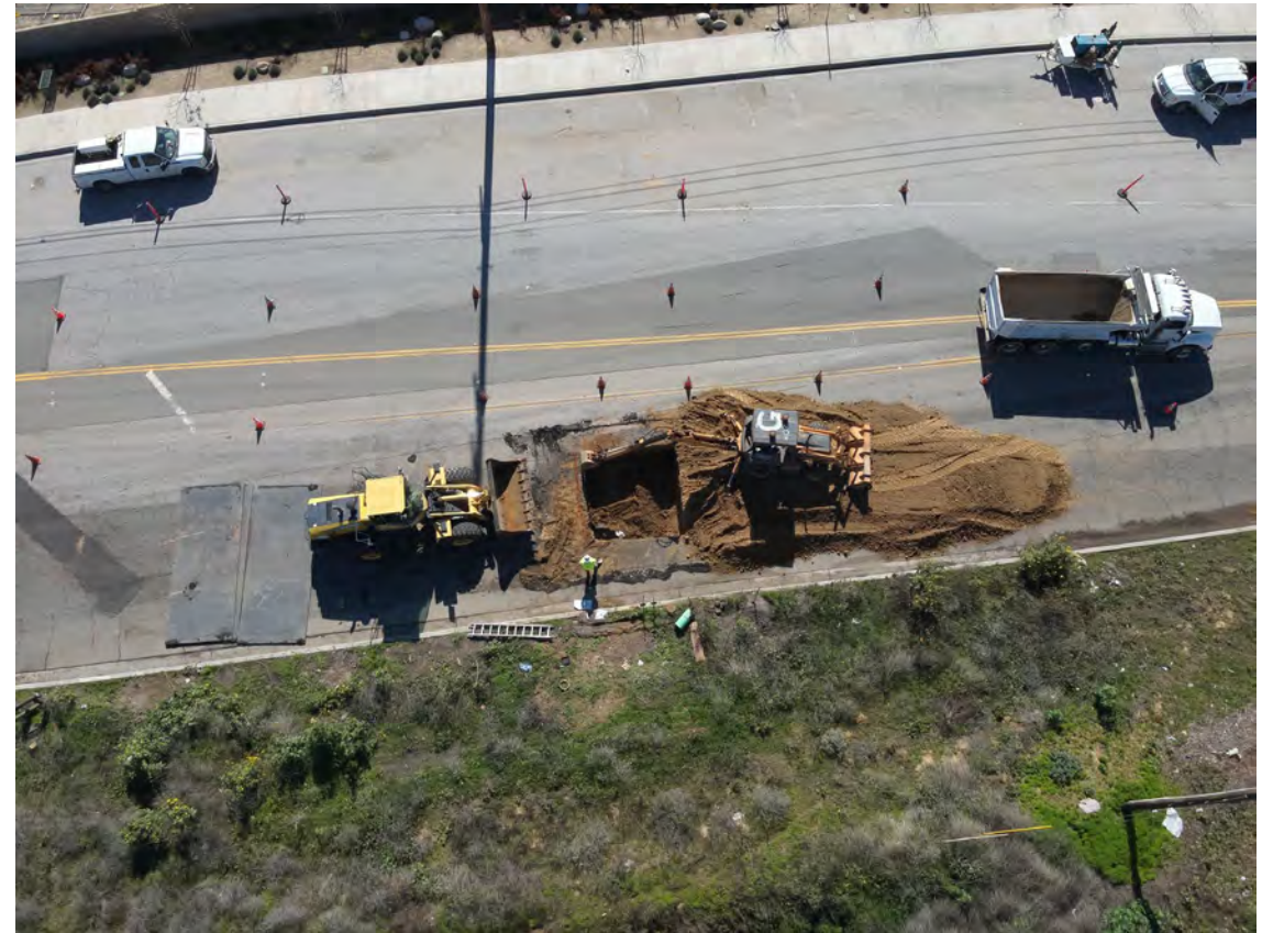
Figure 2: Excavation for tie-in to existing 36" Brine Line.
