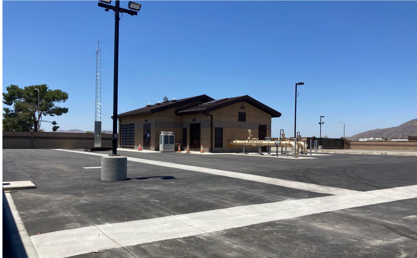
Well 202 Building, July 2023
