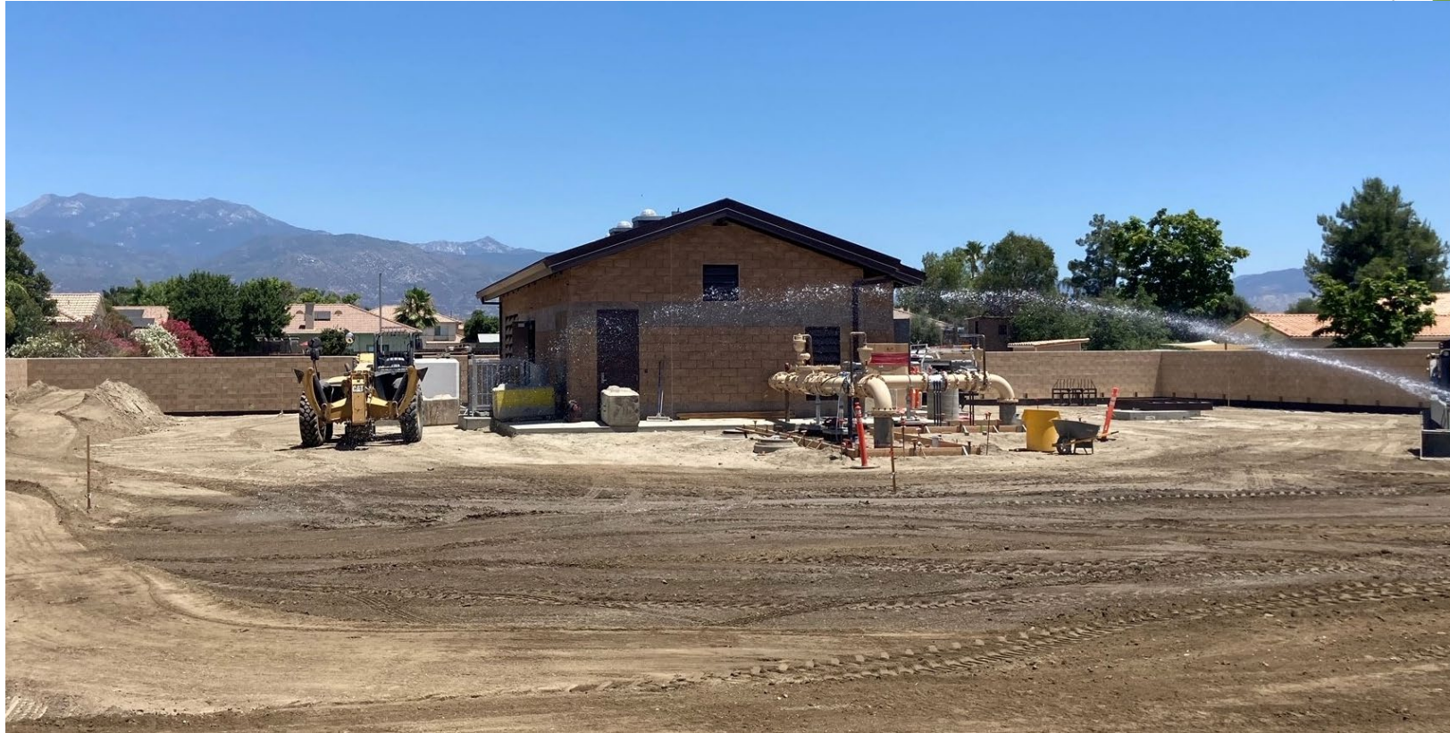
Well 203 Building, July 2023
