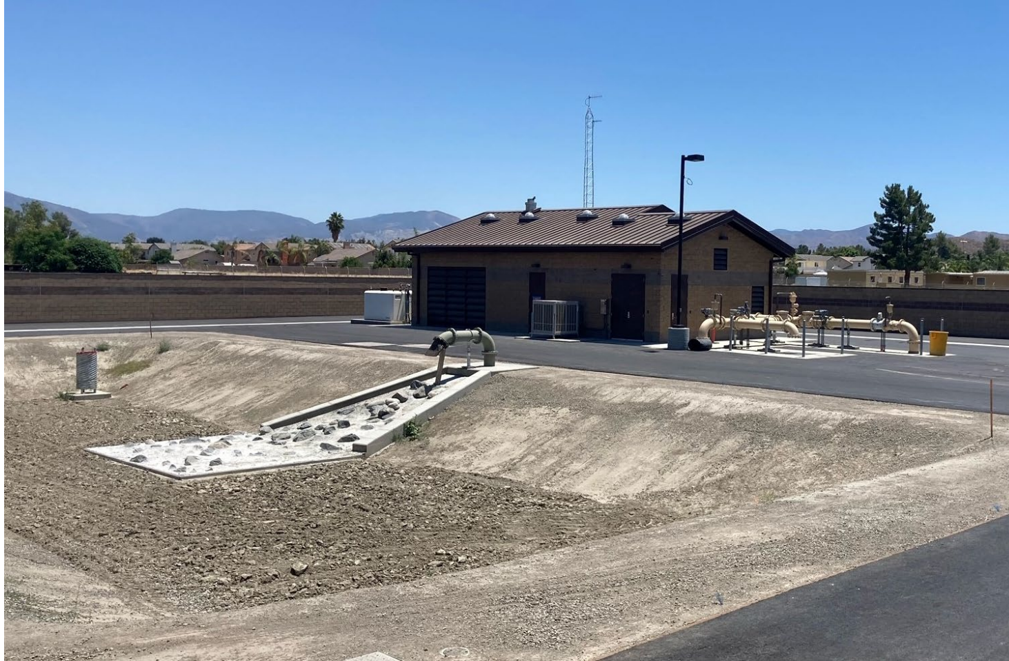
Well 201 Building and Blow Off Pond, July 2023
