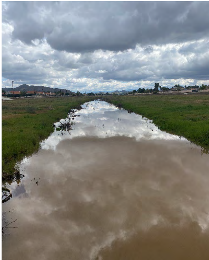
Figure 2-9. Storm Event at Salt Creek at Murrieta Road (March 29, 2022)
