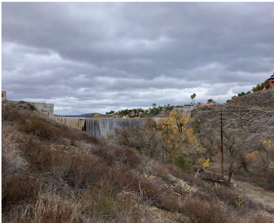
Figure 2-17. Storm Event Sampling Below the Canyon Lake Spillway (December 29-30, 2021)
