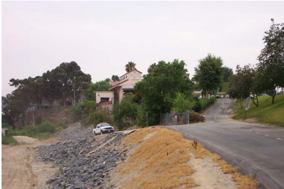
(1) Looking southwest. Car wash building shown in background.
