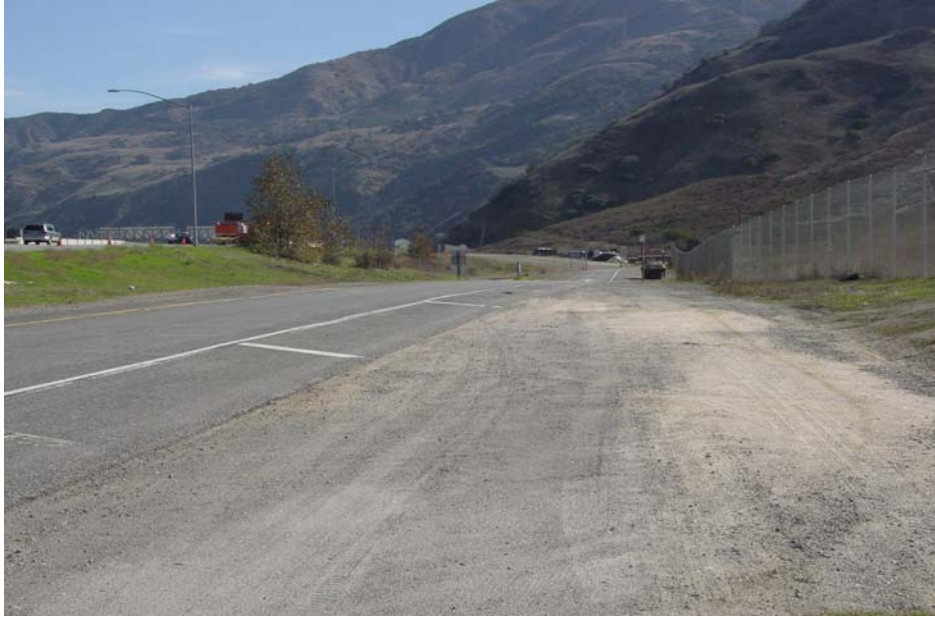
(5A) Looking southeast. View of SR-91 off-ramp at Coal Canyon Road. Access gate is to the left, on north side of SR-91.
