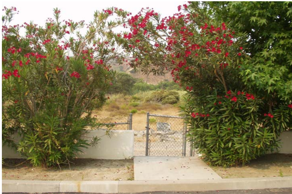
(7) Looking northeast. View of pedestrian access gate leading to SARI Gate structure.
