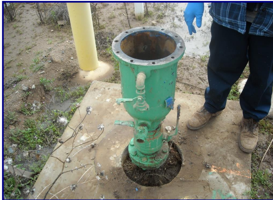
Valve Body with Upper/Lower Ball Valves
