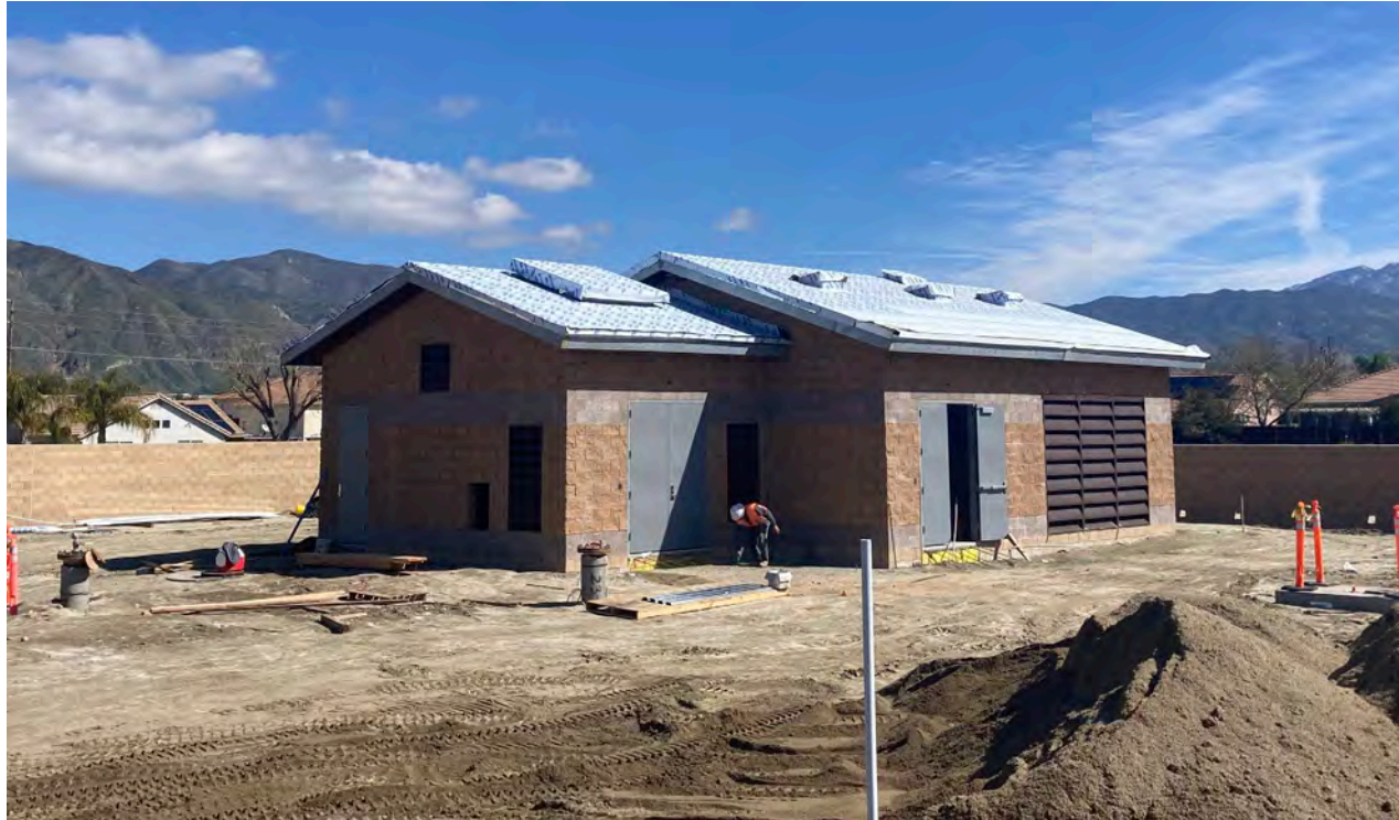
Well 203 Building, March 2023
