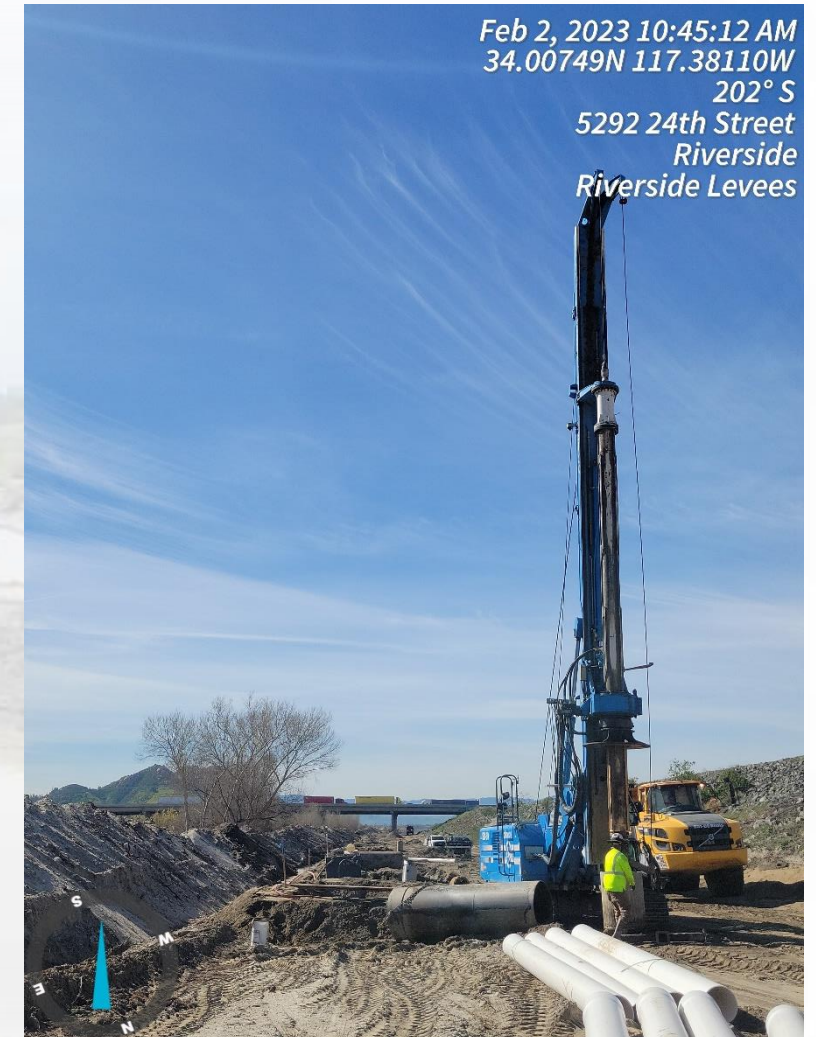
Dewatering Well Installation
