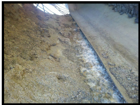
Exposed Concrete Pipe Invert
