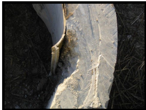
Exposed Concrete Pipe Invert
