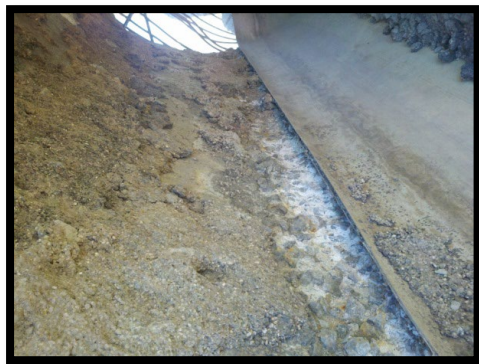
Exposed Concrete Pipe Invert
