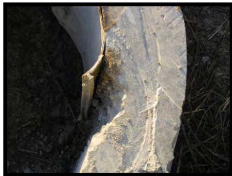
Exposed Concrete Pipe Invert
