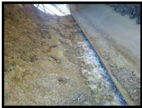
Exposed Concrete Pipe Invert
