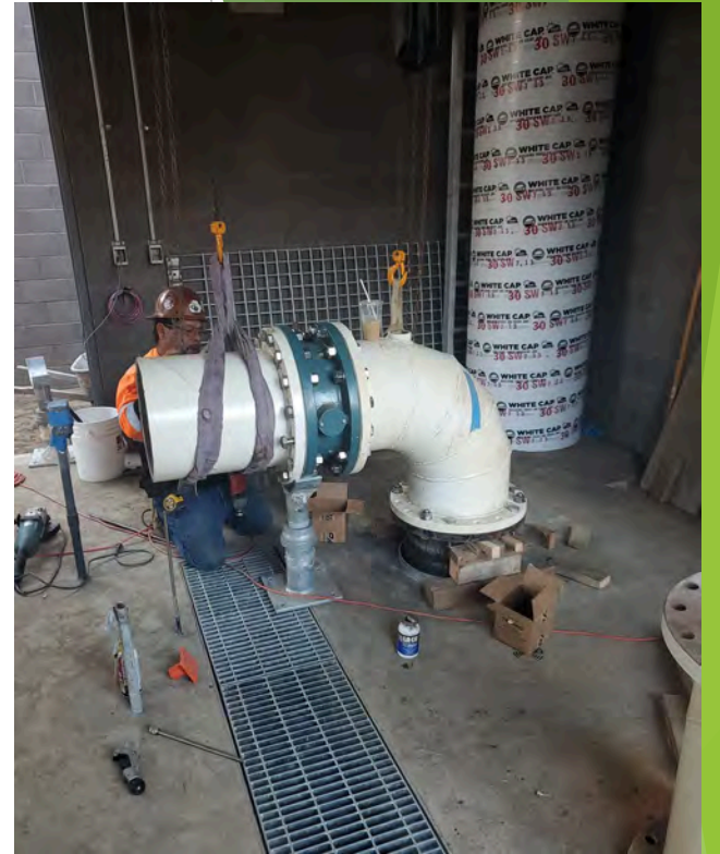
Mesa Well 14 Well Site
