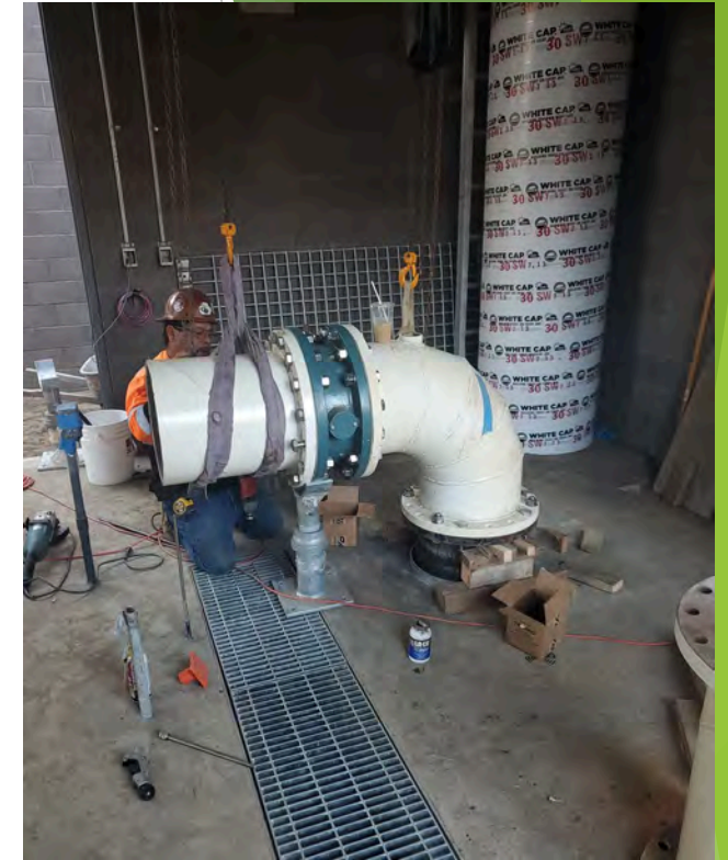
Mesa Well 14 Well Site
