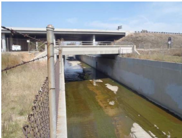
San Antonio Channel @ Walnut Avenue monitoring site.
