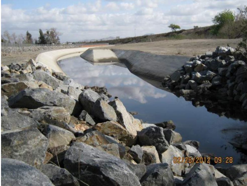
Line E Channel looking upstream.
