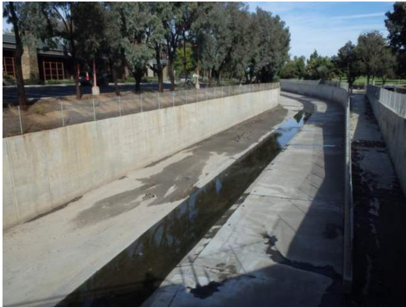
View of Santa Ana Delhi Channel sample site from Irvine Avenue.
