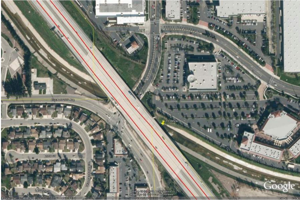
Aerial view of Chino Creek @ Pipeline Avenue monitoring site.
