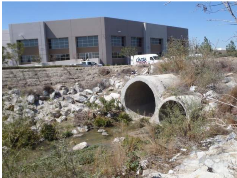
Rialto Storm Drain monitoring site.
