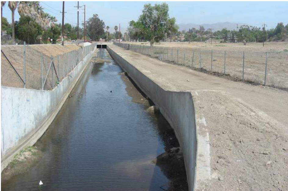
Box Springs Channel looking upstream from Tequesquite Avenue.
