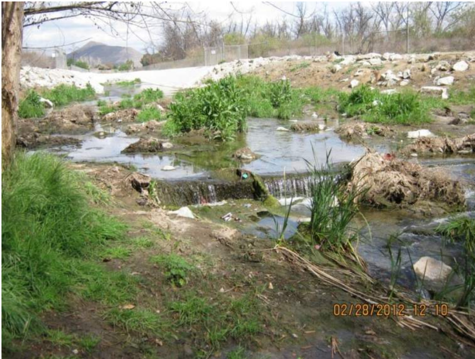
Sunnyslope Channel downstream from transition of lined trapezoidal channel to a channel with natural banks and substrate.
