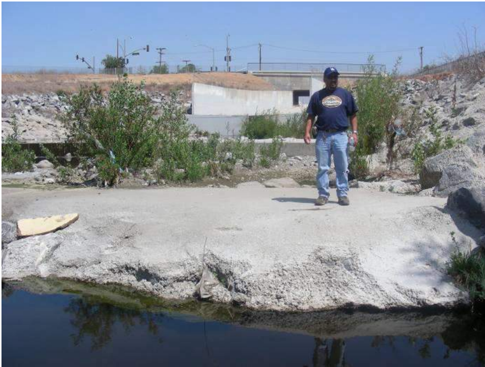
San Sevaine Channel looking upstream from a concrete berm; water in foreground is part of a Santa Ana River backwater area.
