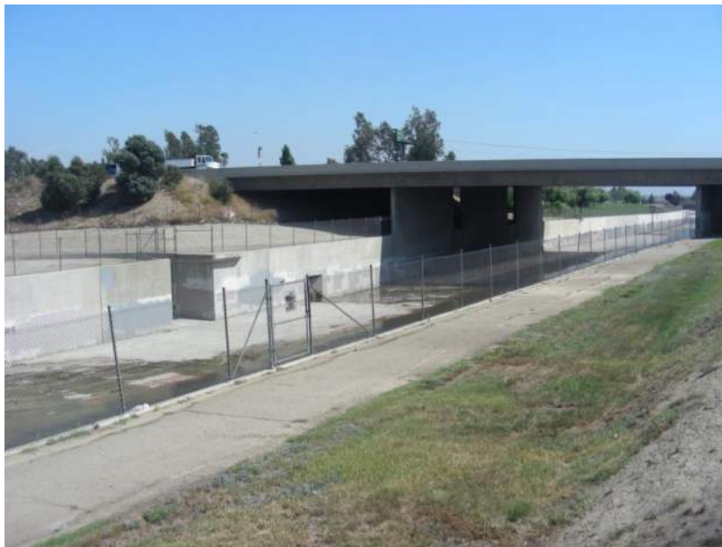
Cucamonga Creek Channel upstream of State Highway 60 monitoring site.
