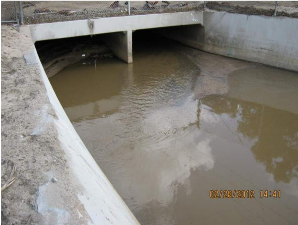
Flowing water on downstream side of Tequesquite Avenue; alternate monitoring site.
