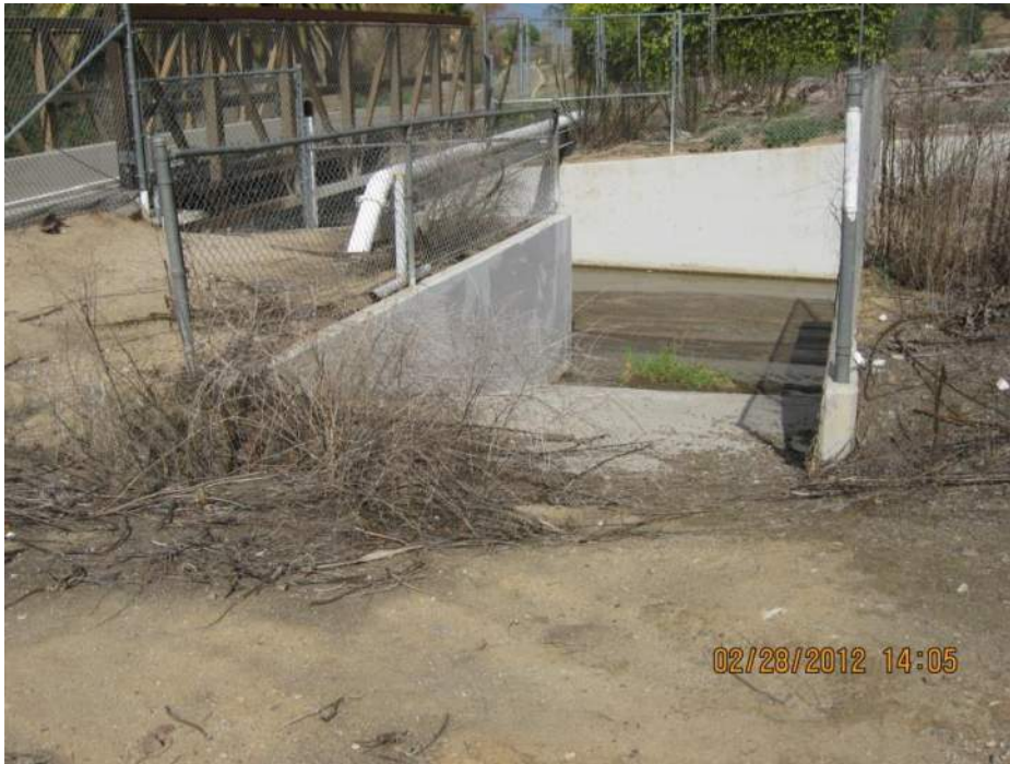
Access ramp into channel.
