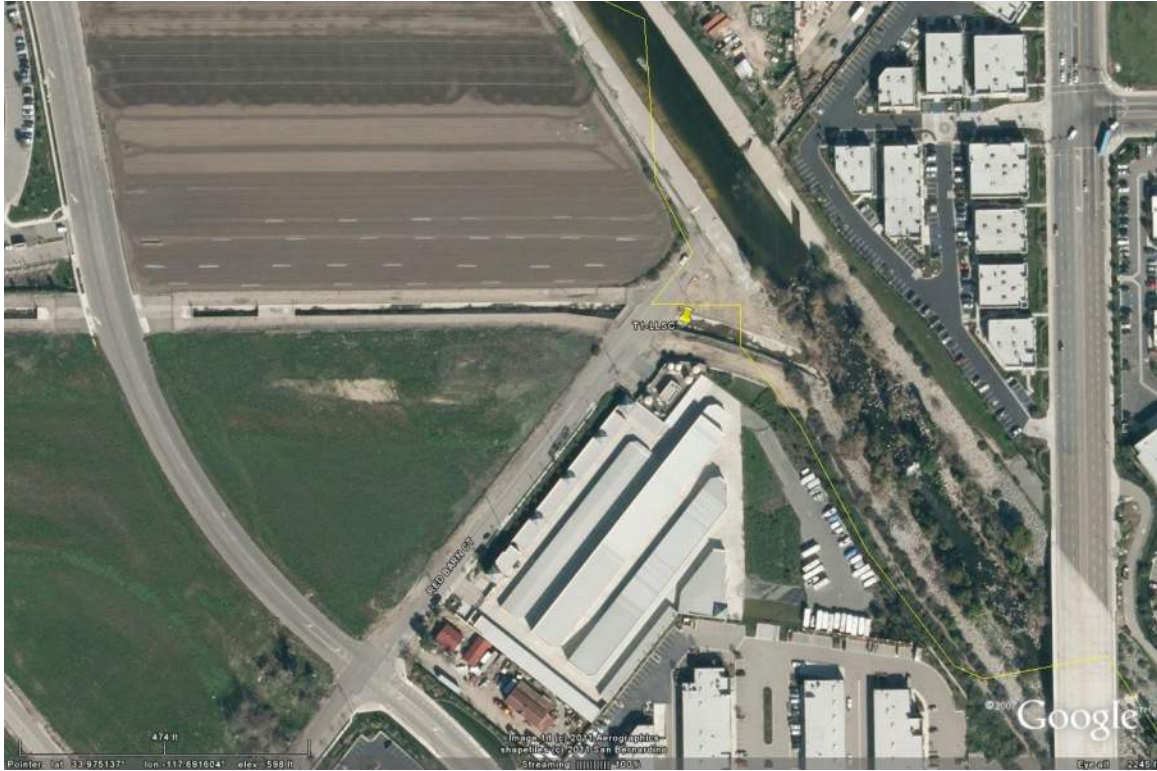
Aerial view of Los Serranos Channel site.
