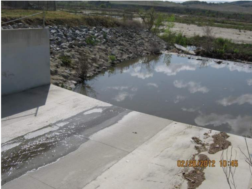
San Sevaine Channel looking downstream.
