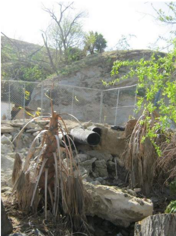
Looking up to outfall pipe location and ongoing construction.
