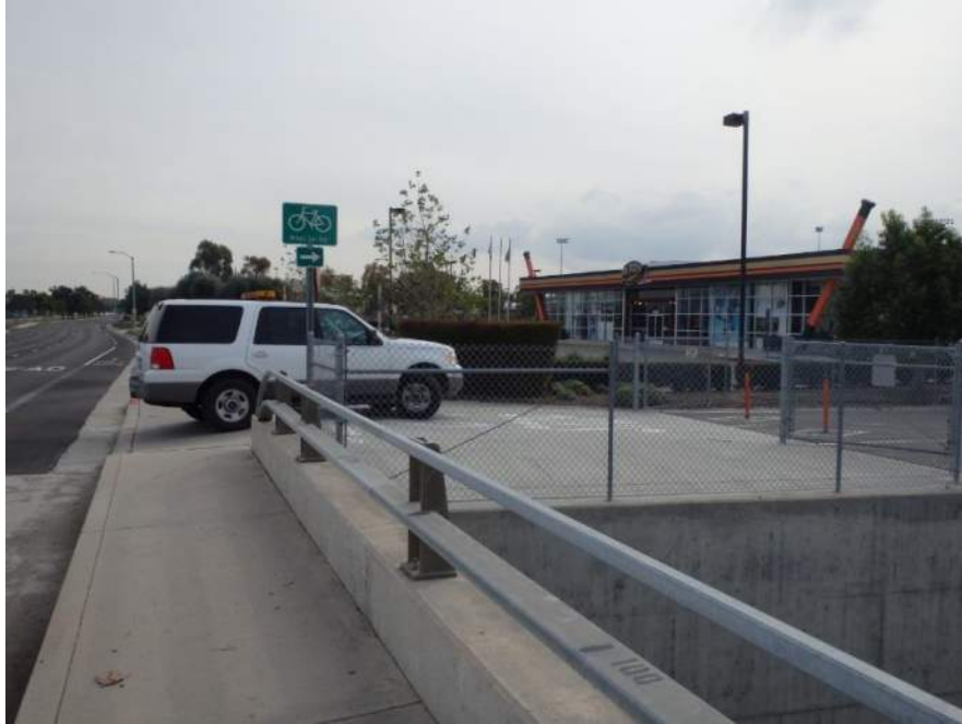
Entry to paved path at Peters Canyon Trail from Barranca Parkway.
