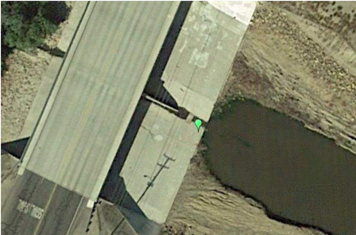
Aerial view of Temescal Creek Reach 1a monitoring site upstream of bridge and downstream of natural bottom section.
