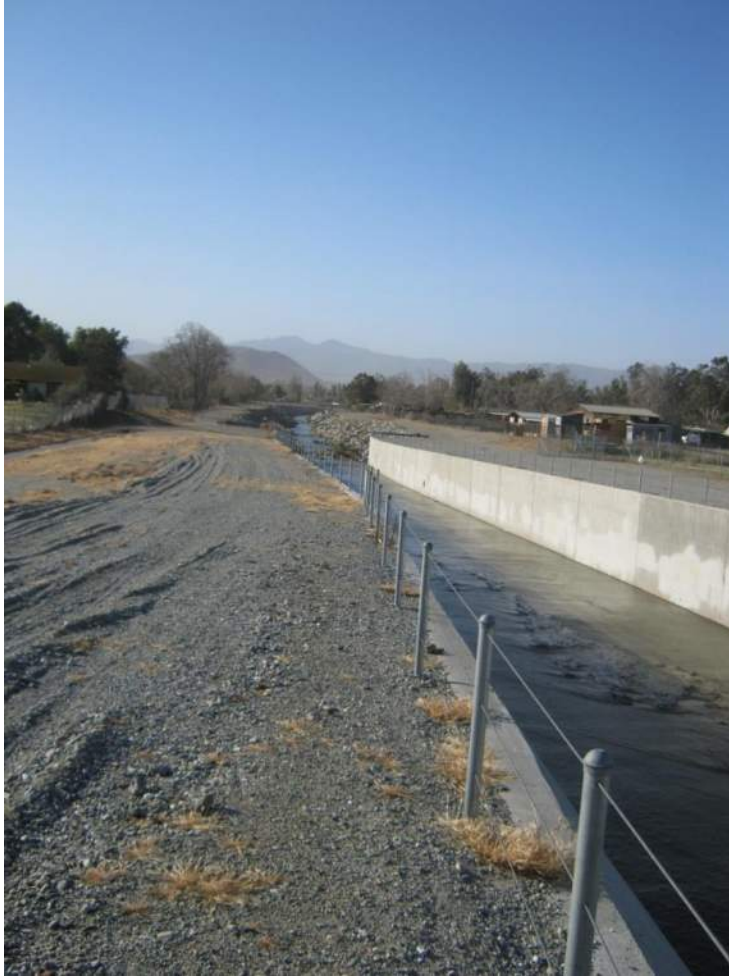
View of Day Creek looking downstream toward future construction area.
