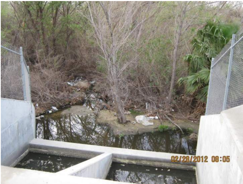
Outfall looking downstream.
