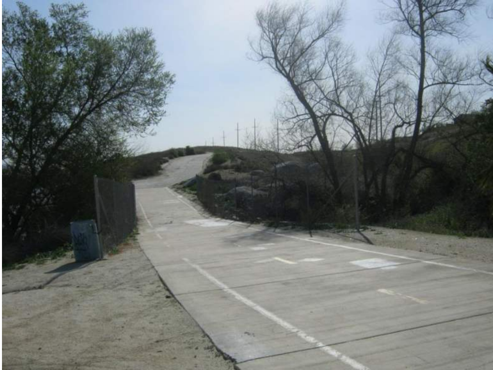
Bike path bridge crossing over drainage area.
