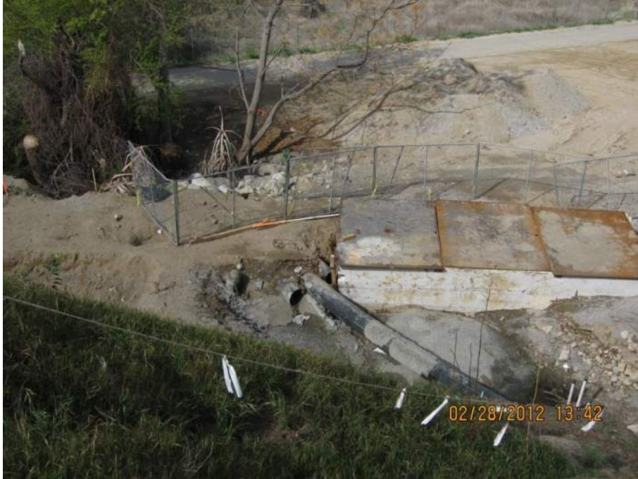
View of ongoing construction and new monitoring site.
