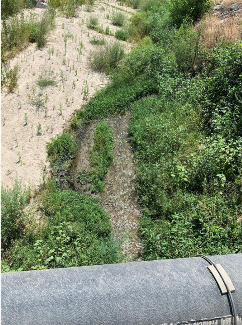
View of San Timoteo Creek Reach 3 below Live Oak Canyon Rd bridge
