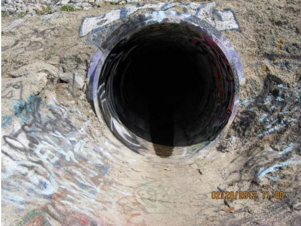
Looking up into outfall pipe.
