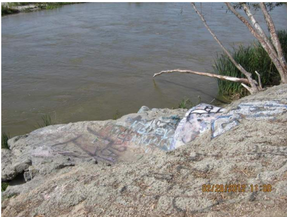
Outfall structure on the Santa Ana River.
