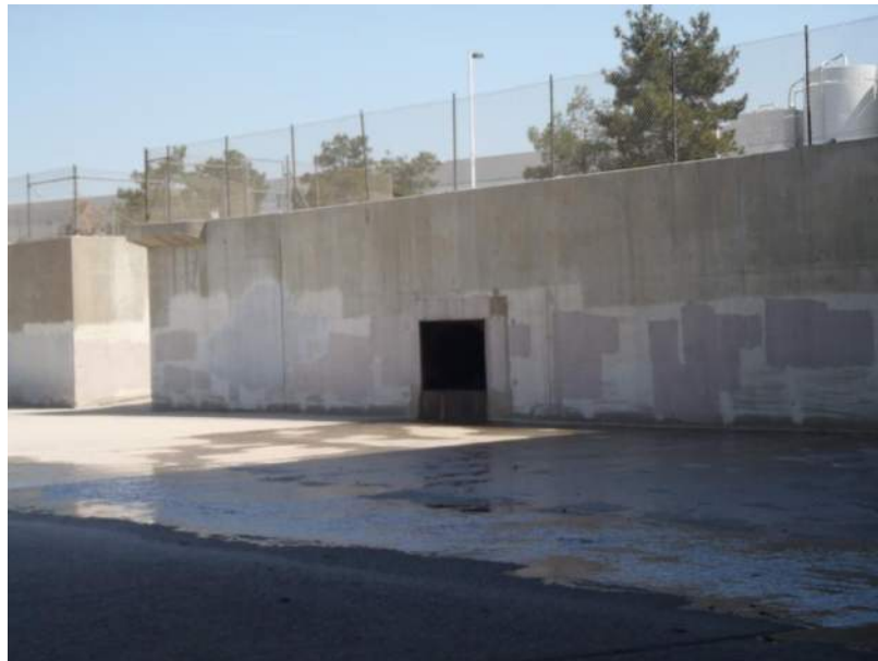
Chris Basin (Lower Deer Creek Channel) monitoring site.
