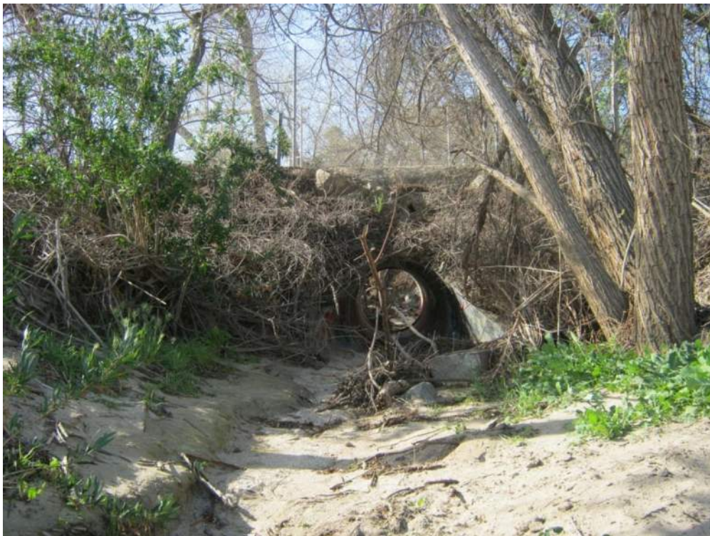
Culvert pipe underneath bike path.
