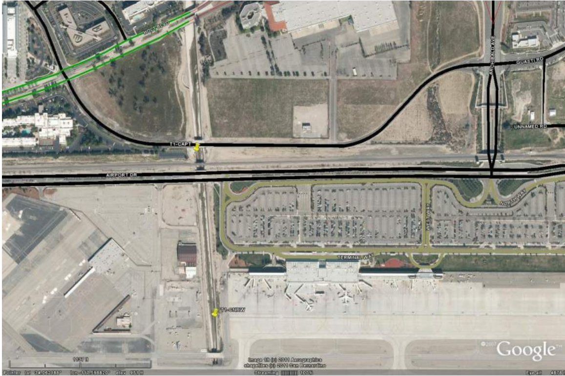
Aerial view of Airport Drive @ Cucamonga Creek Channel.
