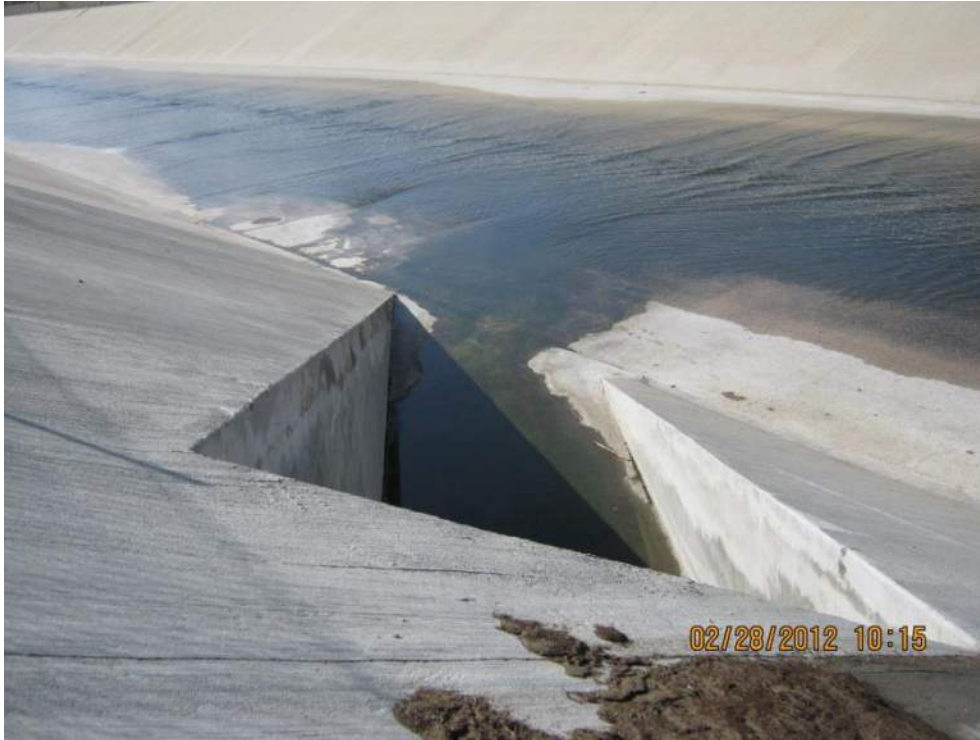
Looking downstream from outfall structure.
