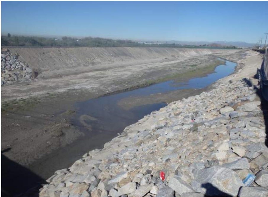
Looking upstream at Bolsa Chica Channel from access gate. Channel runs parallel to Bolsa Chica Rd here.
