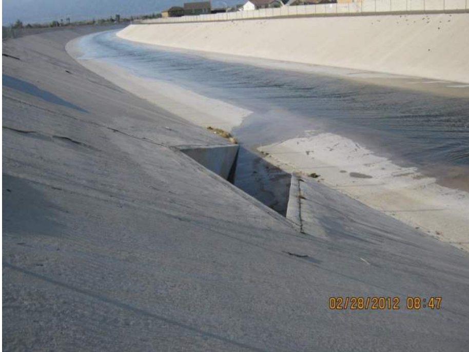
Looking downstream from outfall structure.
