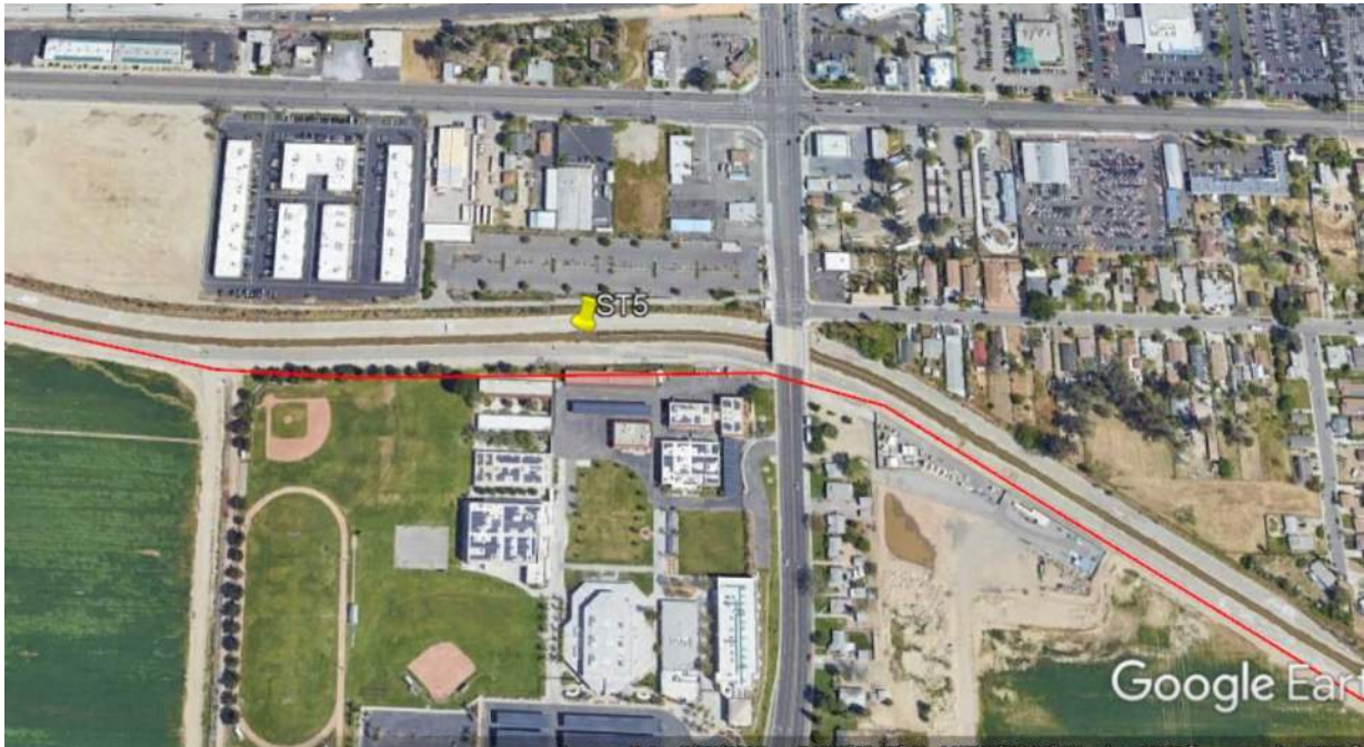
Aerial view of monitoring site on San Timoteo creek west of Anderson street crossing
