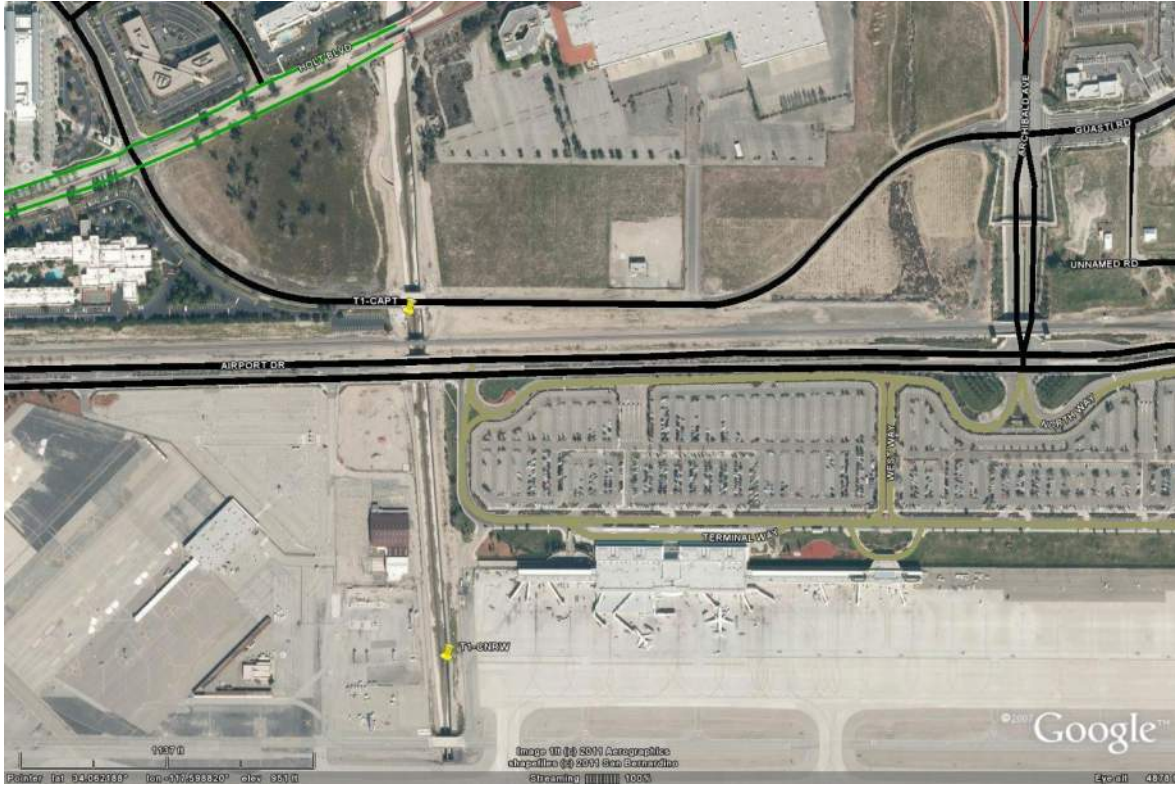
Aerial view of North Runway @ Cucamonga Creek Channel.
