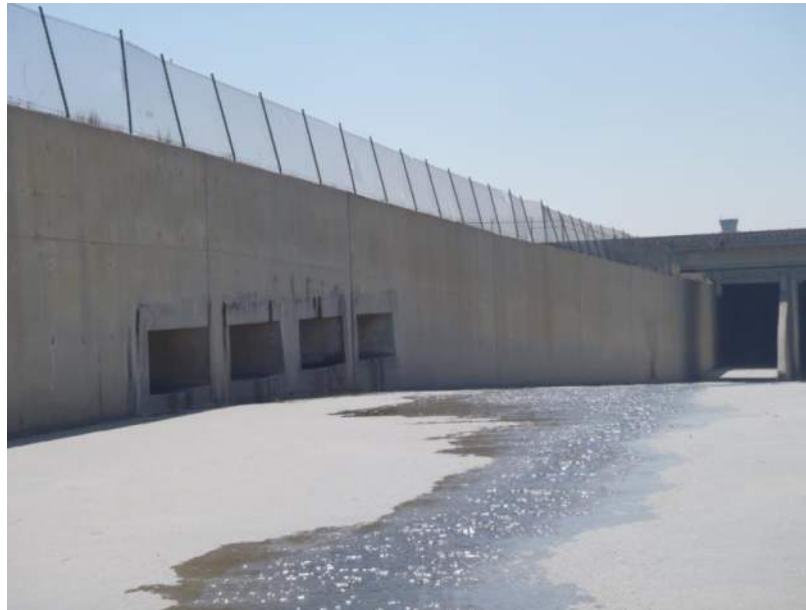
North Runway @ Cucamonga Creek Channel monitoring site.
