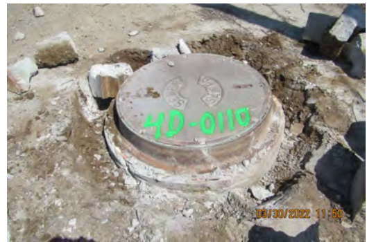
Removal of concrete collar around MAS on Reach IVD
