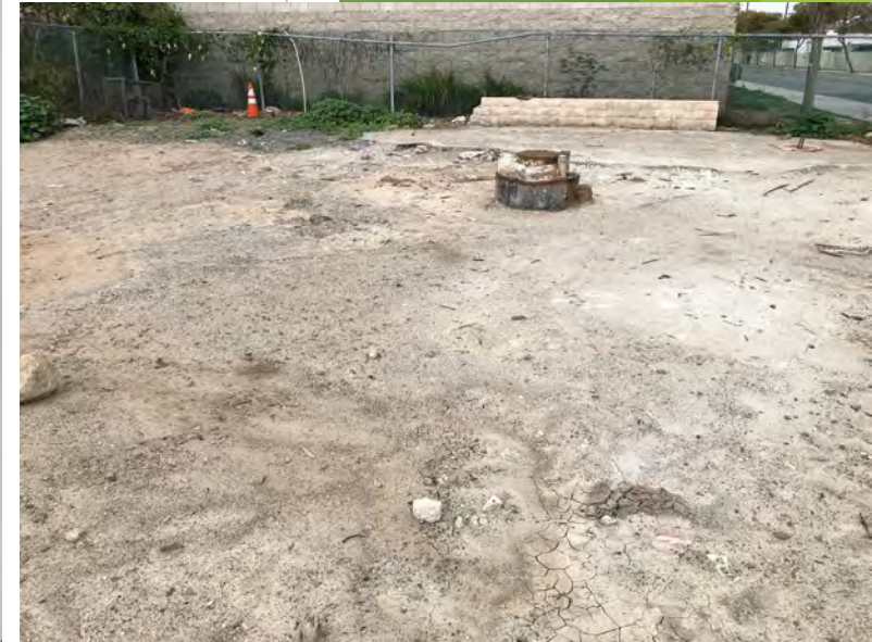
Well construction completed
