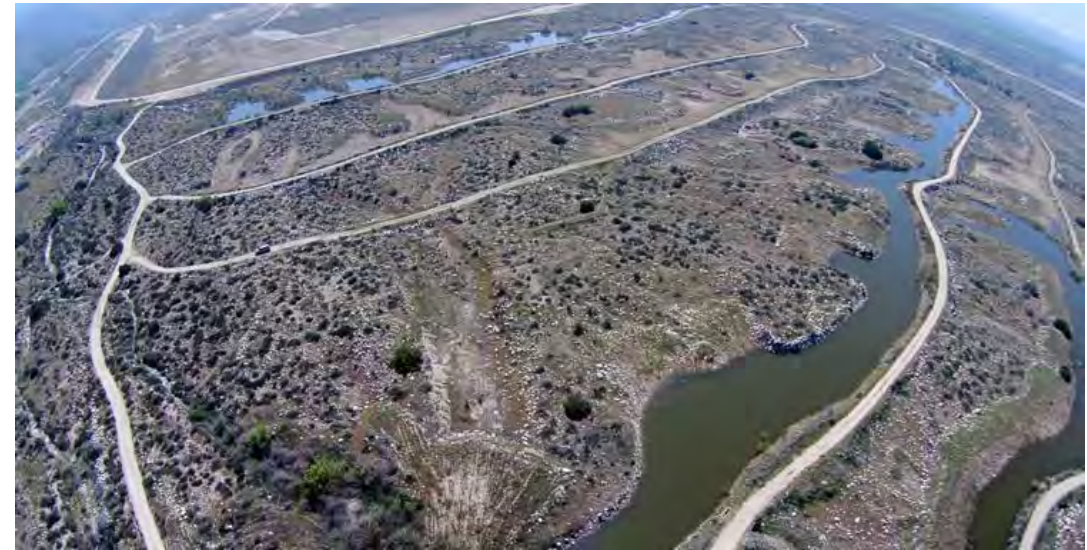
SBVWCD Recharge Facilities
