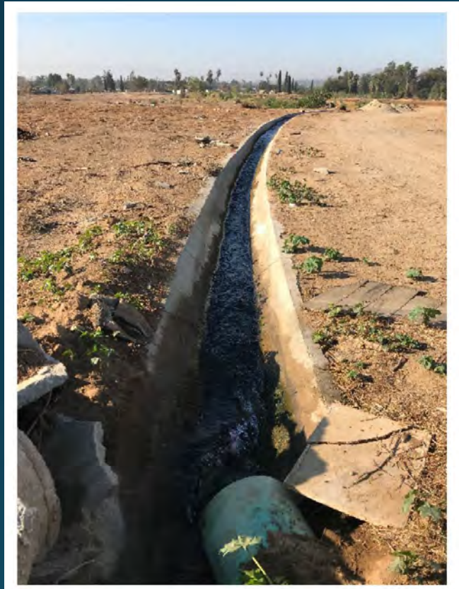
WSC Photo: Jurupa Ditch transitioning from pipe to open ditch.
