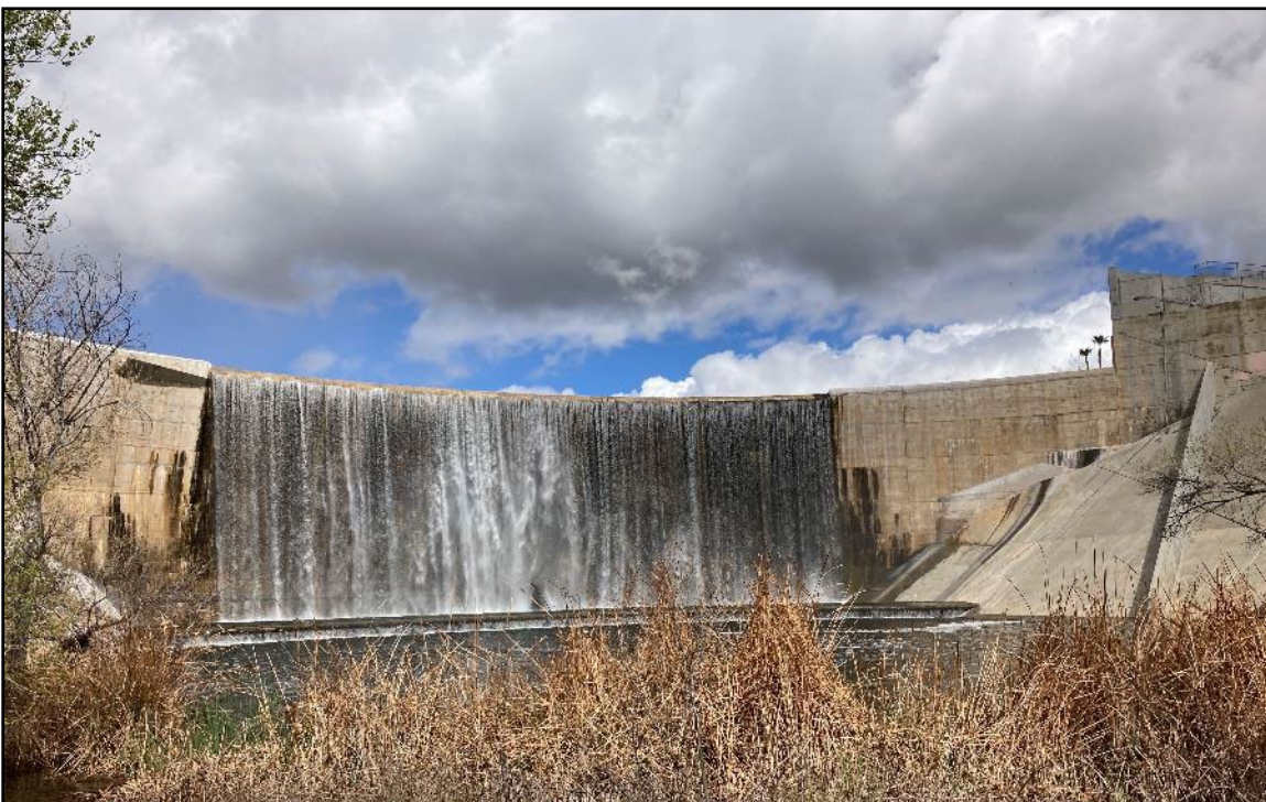
Figure 2-16. Canyon Lake Spillway (March 10 - 15, 2021)
