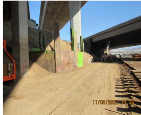
Reach V / IVB contractor coordination
