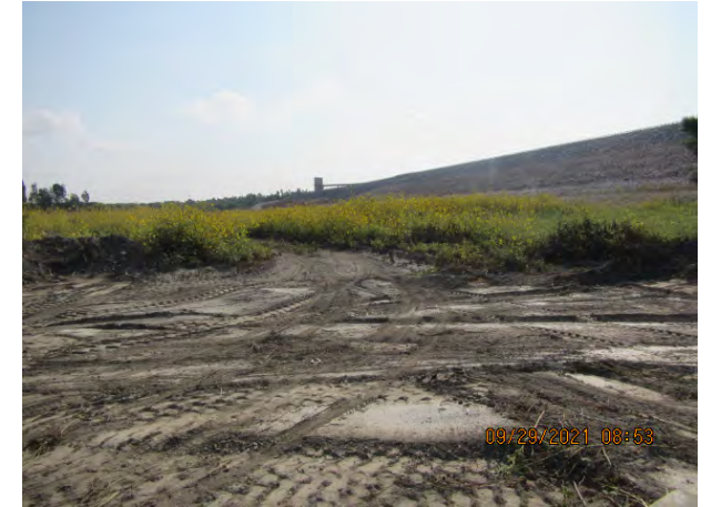
Reach IVA / IVB ROW clearing - Prado
