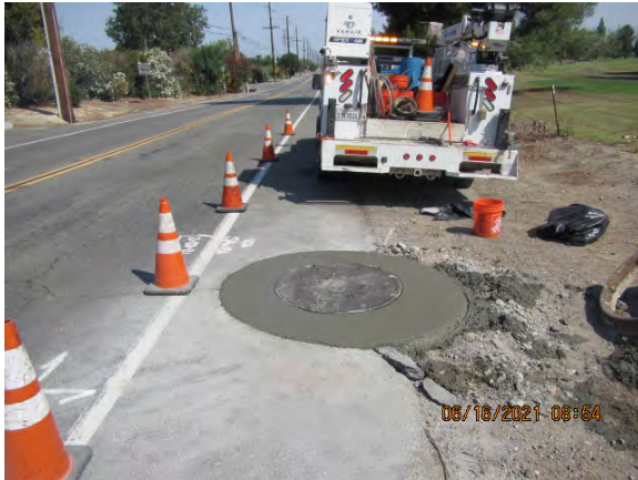
Reach IVA MAS inspections / repairs / corrosion protection
