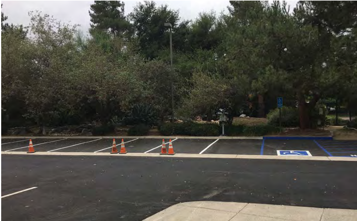
E3 PHOTO E3- Existing Accessible Parking; Non-compliant Path of Travel
