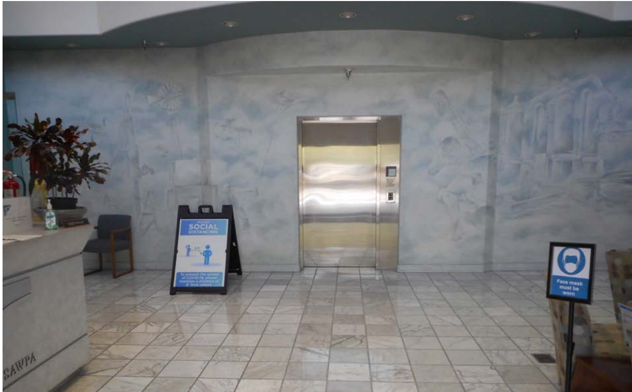
C1 PHOTO C1 - Existing Mural at Lobby
