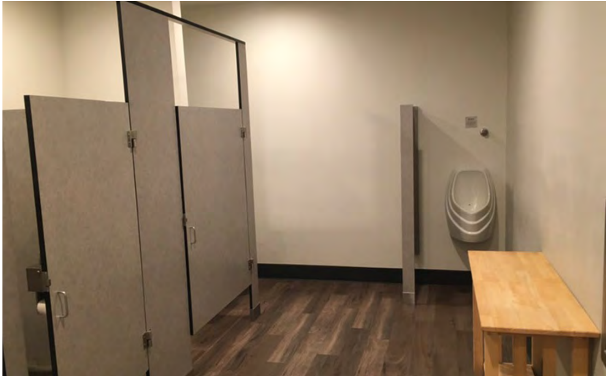
J2 PHOTO J2- Existing Urinal at Men's Restroom | First Floor
