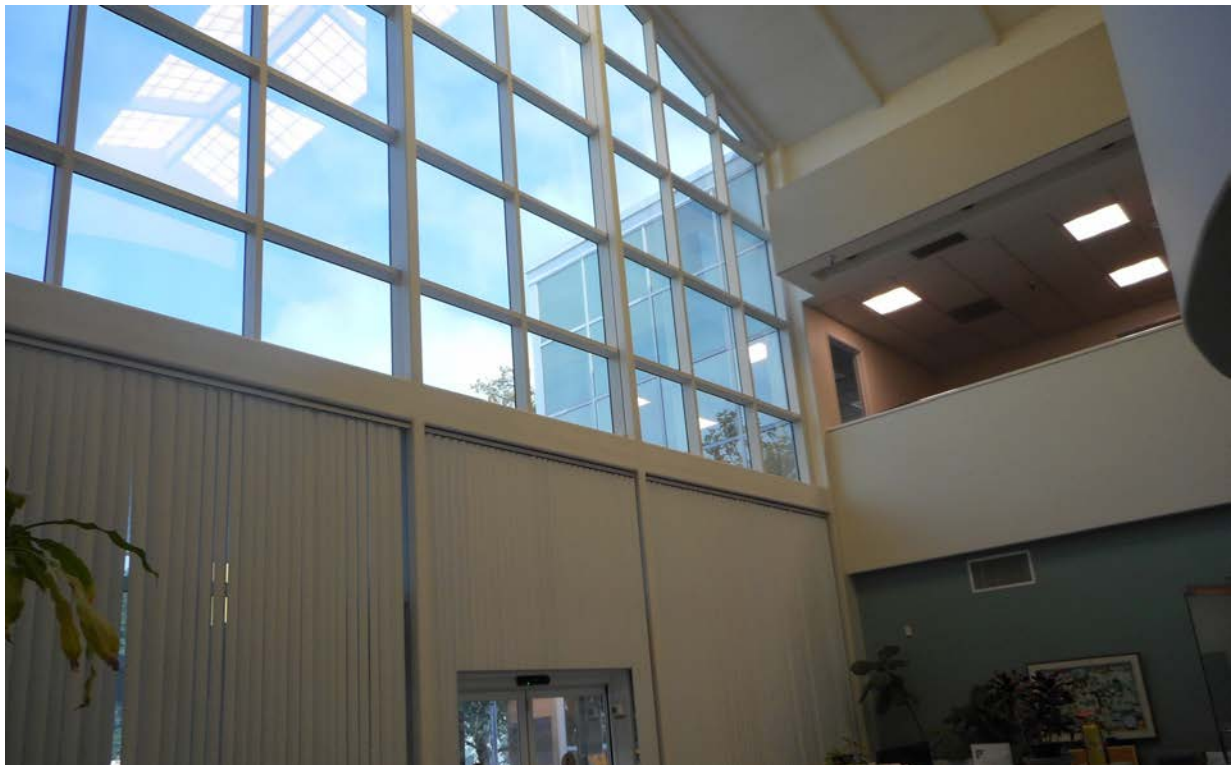
B1 PHOTO B1- Existing Window Treatment
