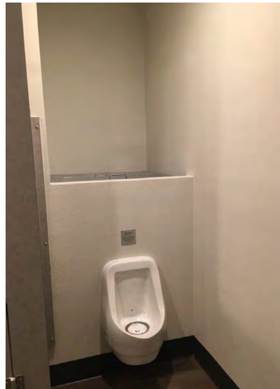
I2 PHOTO I2- Existing Urinal at Men's Restroom | First Floor
