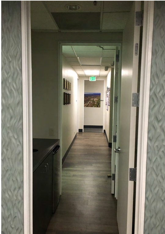
A3 PHOTO A3- Existing Vestibule (Potential Door Maneuvering Issues)
