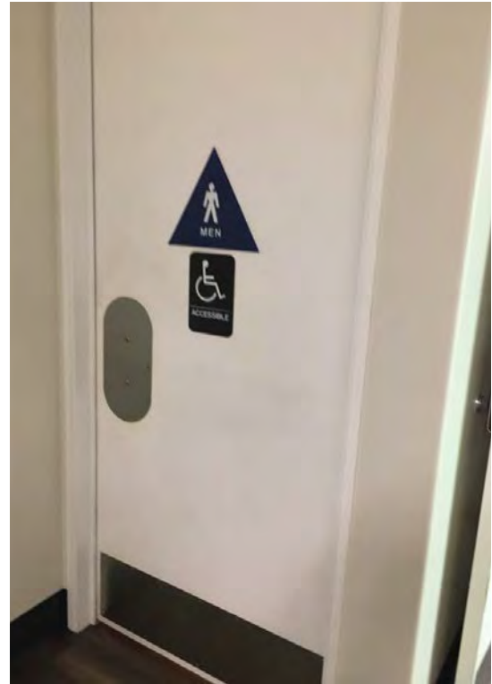
G2 PHOTO G2- Existing Men's Restroom Door & Signage
