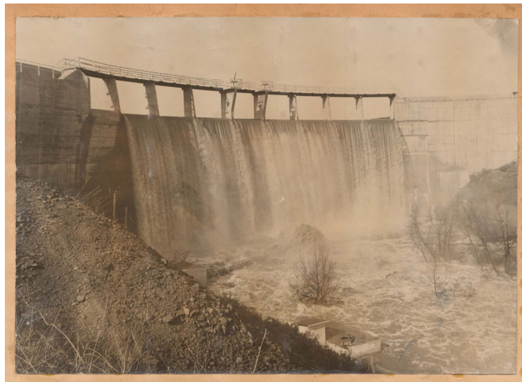
Figure 2-12. Overflow of Canyon Lake Dam, approximately 1936-1937 (Source: Lake Elsinore Naval School)
