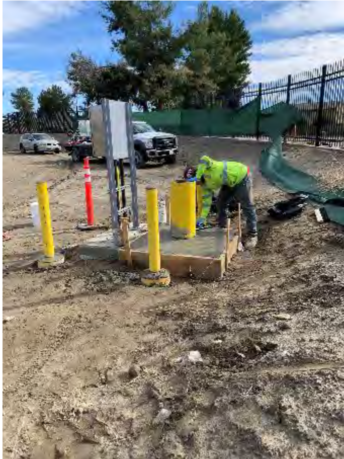
Shallow Monitoring Well SW-06
