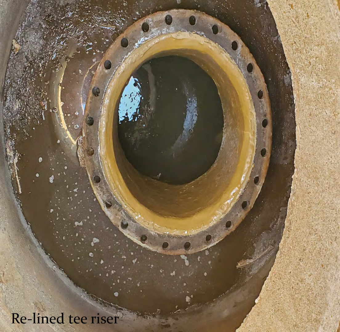
Metal filler used for flange lip
