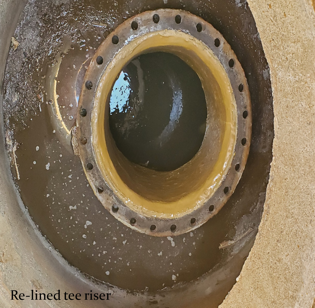
Metal filler used for flange lip
