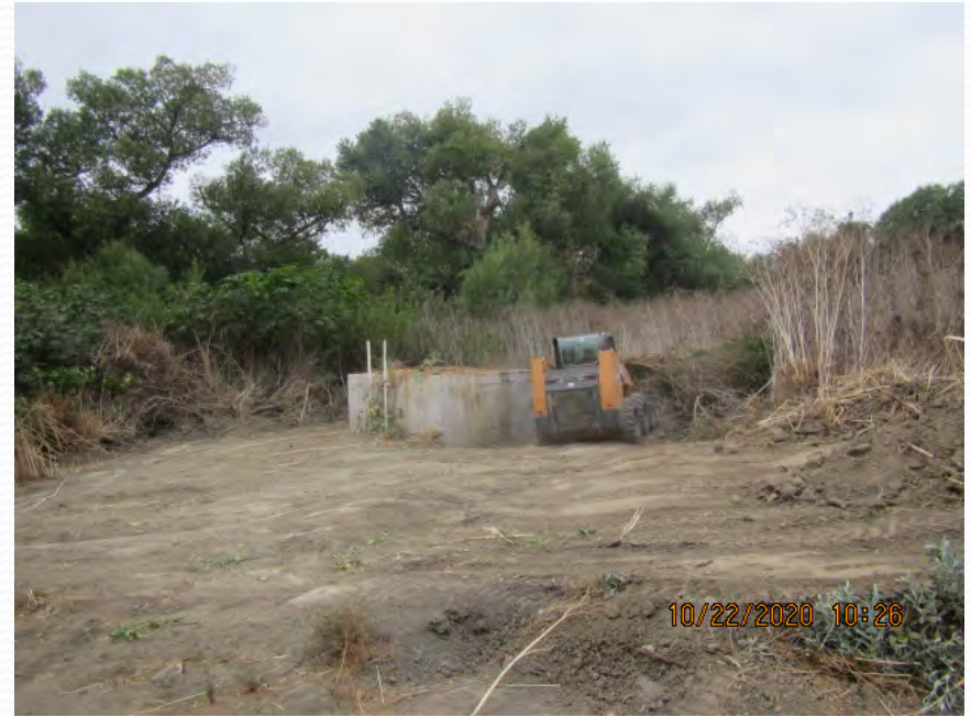
Upstream Maintenance Access Structure
