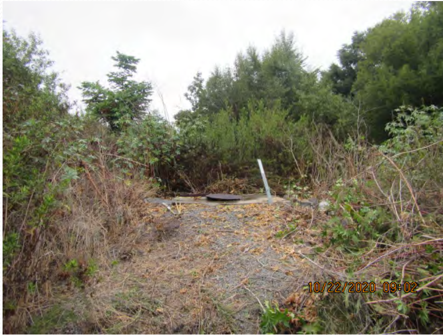
Downstream Maintenance Access Structure
