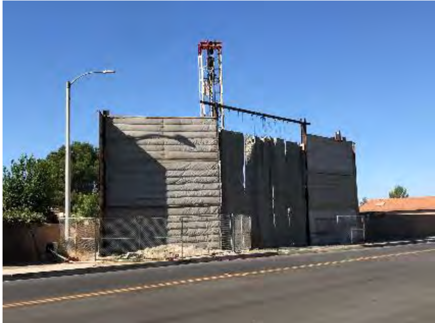
Drill Rig and Sound Walls
