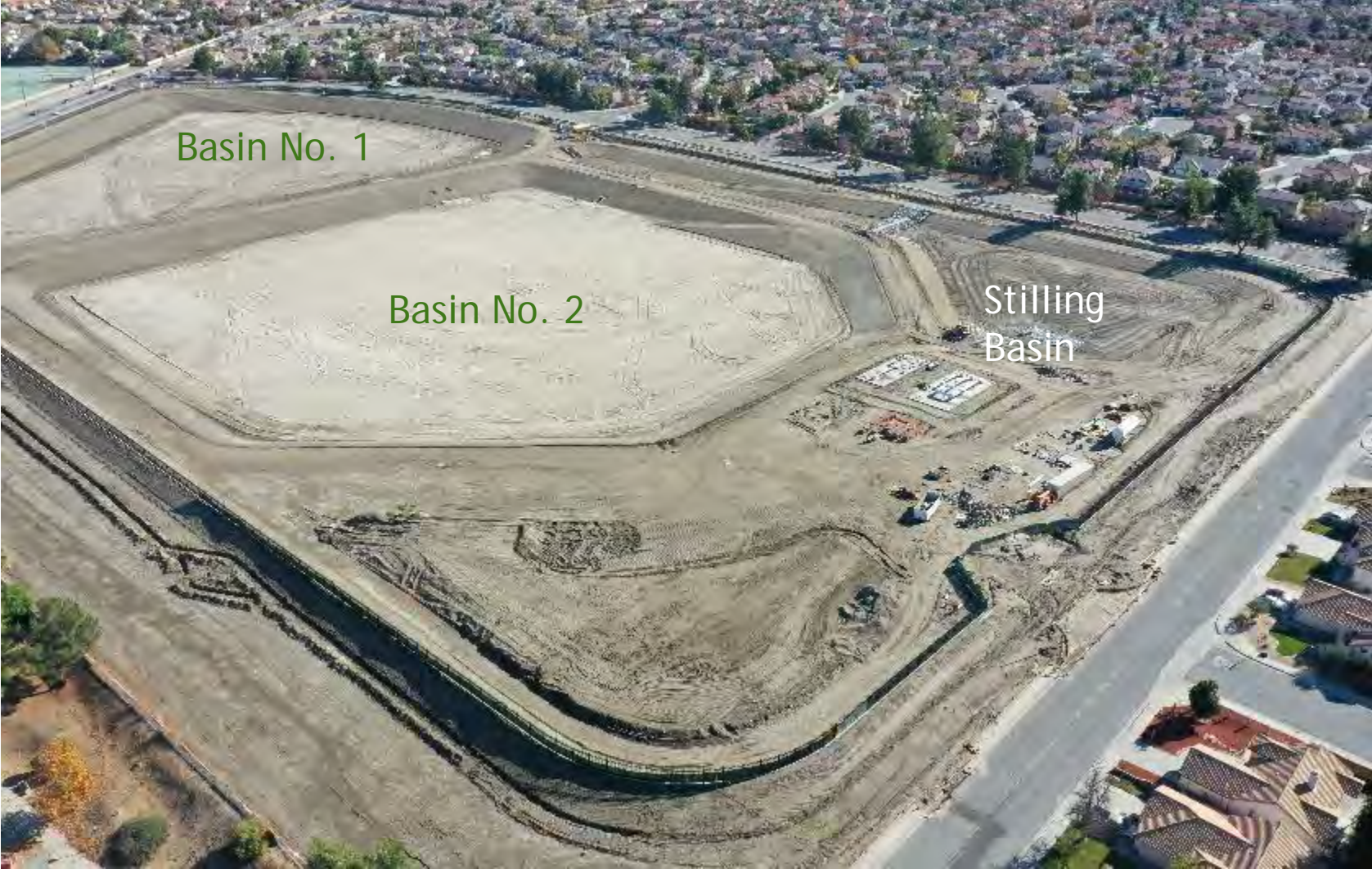
Aerial Site View
