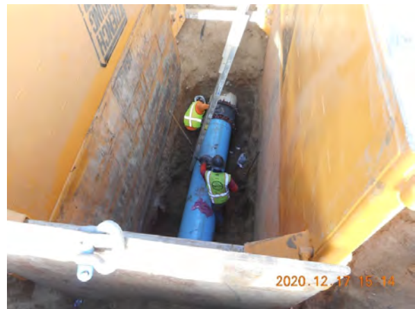
Figure 3. Repaired Pipe.
