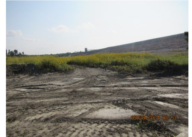
Reach IVA / IVB ROW clearing - Prado
