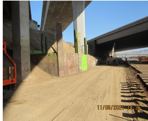
Reach V / IVB contractor coordination
