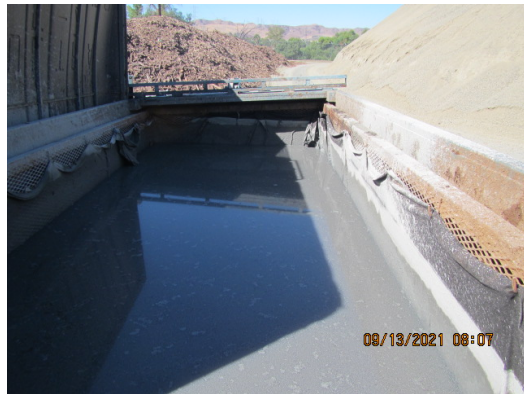
Reach IVA line cleaning / debris disposal
