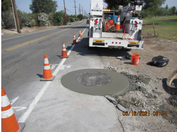
Reach IVA MAS inspections / repairs / corrosion protection
