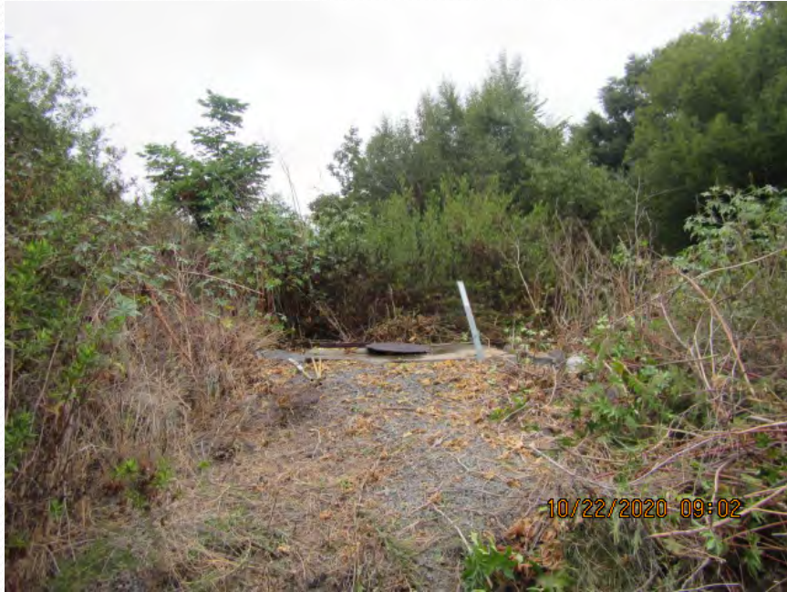
Downstream Maintenance Access Structure
