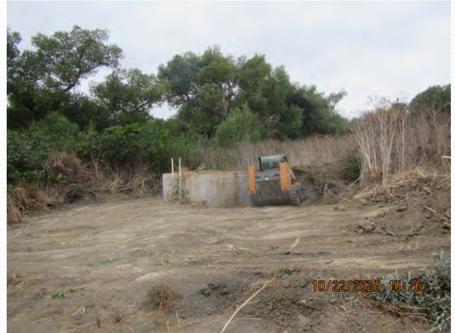
Upstream Maintenance Access Structure
