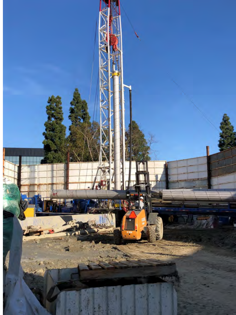
Casing installation
