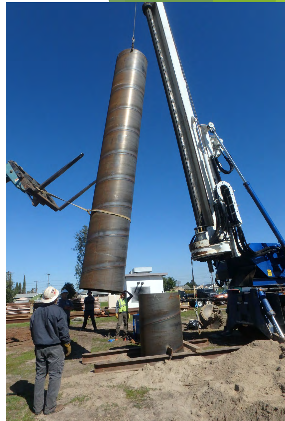
Sanitary seal installation
