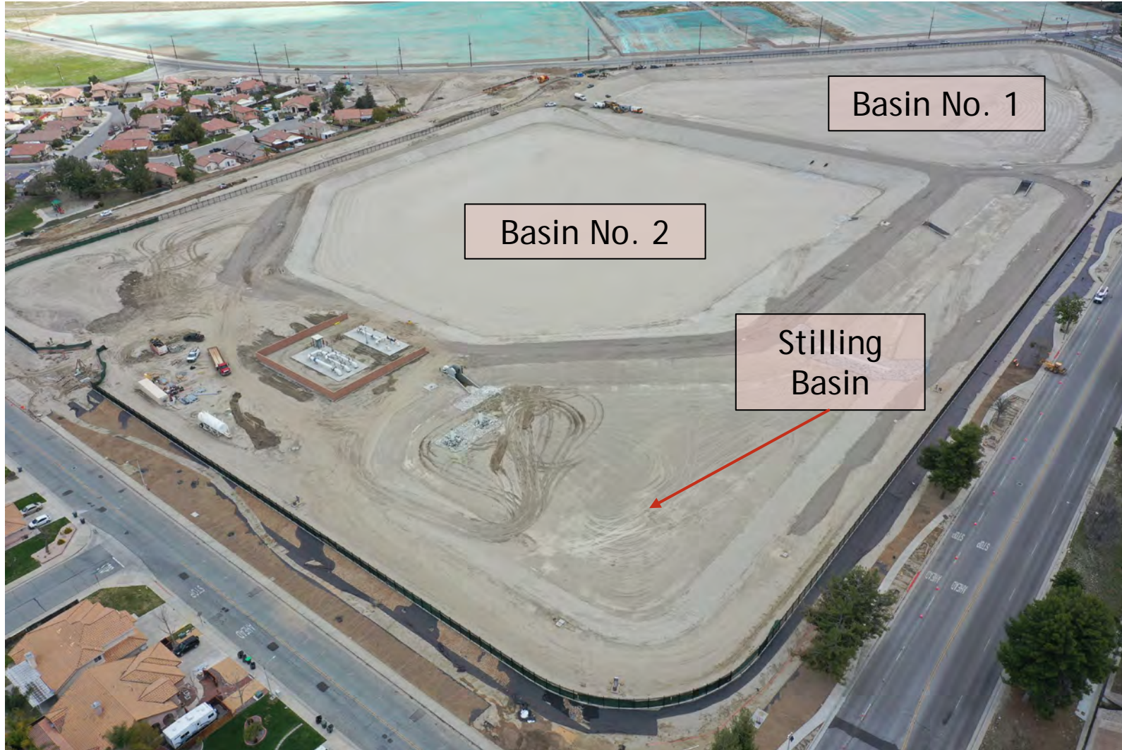
Aerial Site View
