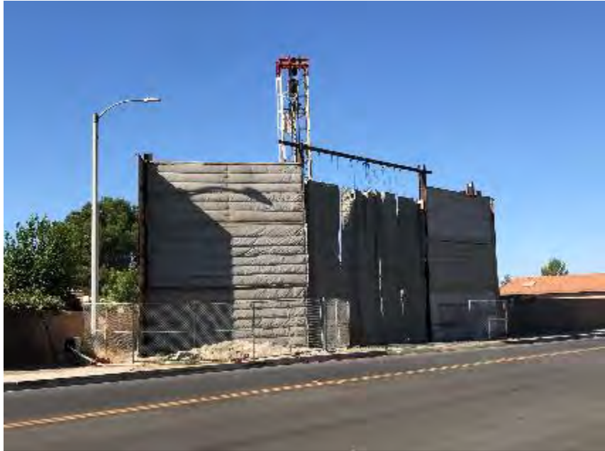
Drill Rig and Sound Walls
