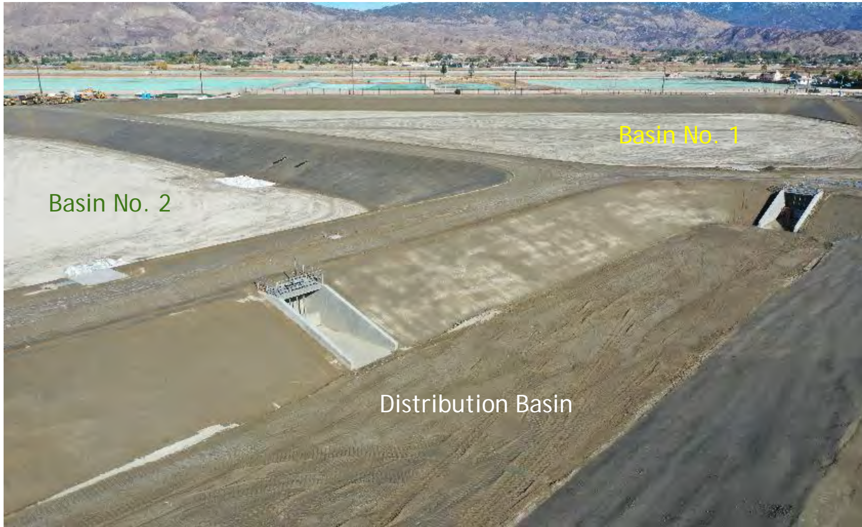
Distribution Basin and Outlet Control Facilities
