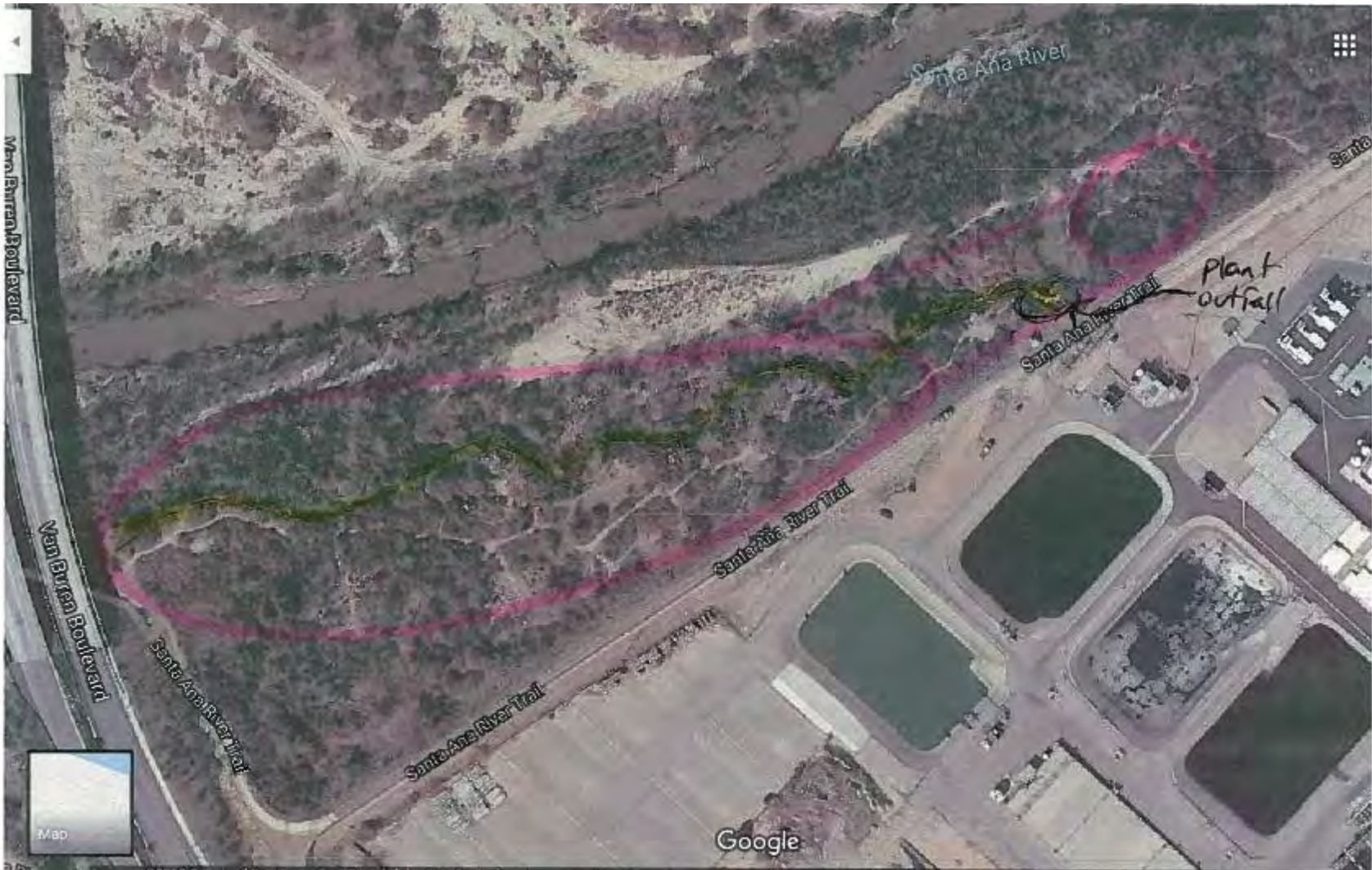
Figure 2-20. Homeless Encampments in the Santa Ana Riverbed along Riverside RWQCP Upstream of the Van Bureau Boulevard Bridge. Note location of Plant's Effluent Outfall (Image courtesy of Ed Filadelfia, City of Riverside, Public Works, Sewer Systems)
