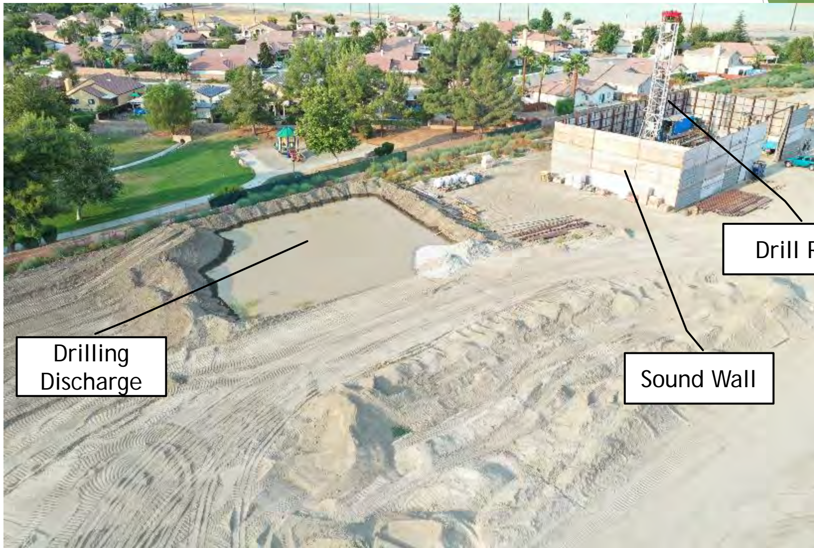
Construction of a Monitoring Well at Mountain Avenue West Recharge Facility
