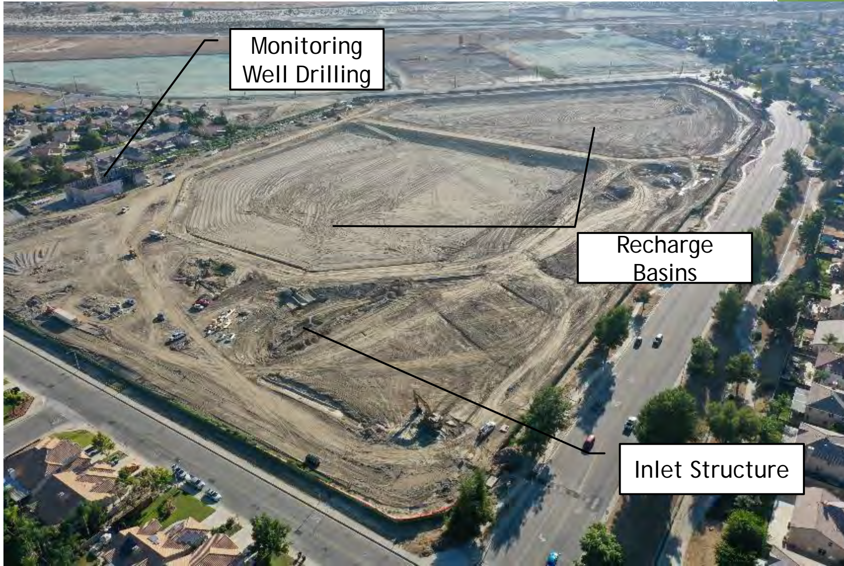
Recharge Basin Construction
