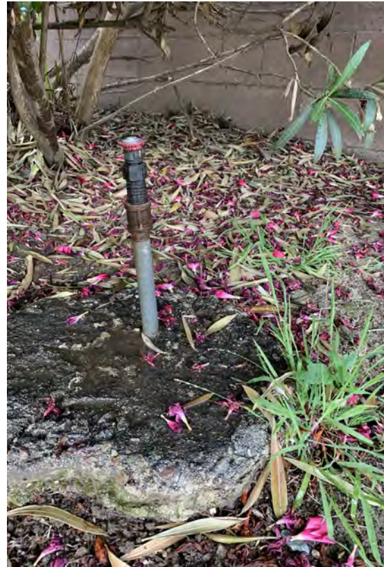
Irrigation "Tune-Up" Sprinkler Head Fixed
