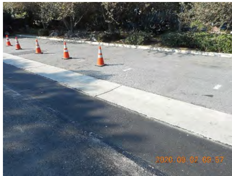
Figure 1. West side of the SAWPA Parking Lot. The contractor completed the over-excavation adjacent to the gutter to ensure a minimum asphalt thickness of 3 inches.
