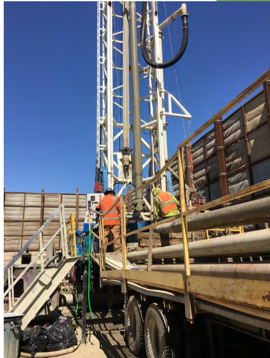
Construction of a Monitoring Well at Mountain Avenue West Recharge Facility
