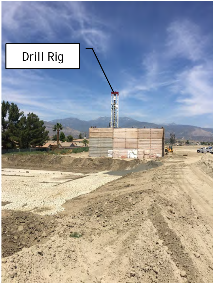
Construction of a Monitoring Well at Mountain Avenue West Recharge Facility
