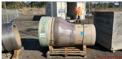
Upstream connection to existing 27" Reinforced Concrete Pipe and downstream connection to existing 36" fiberglass reinforced pipe.
