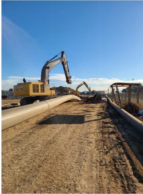
Installation of new HDPE pipe.
