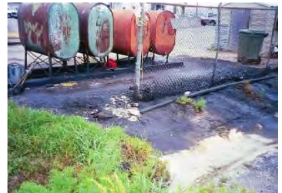
Pollution Control Inspection Point
